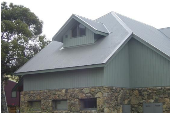
Figure – Example of rooms within the roof space
