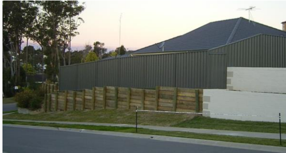
Example of retaining walls and fencing that is not permitted on corner lots.
