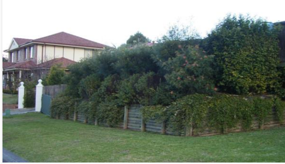
Example of stepped retaining walls and landscaping to screen fencing on corner lots
