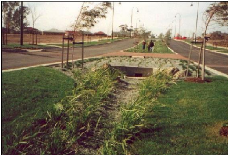
Road network and grass swales.
