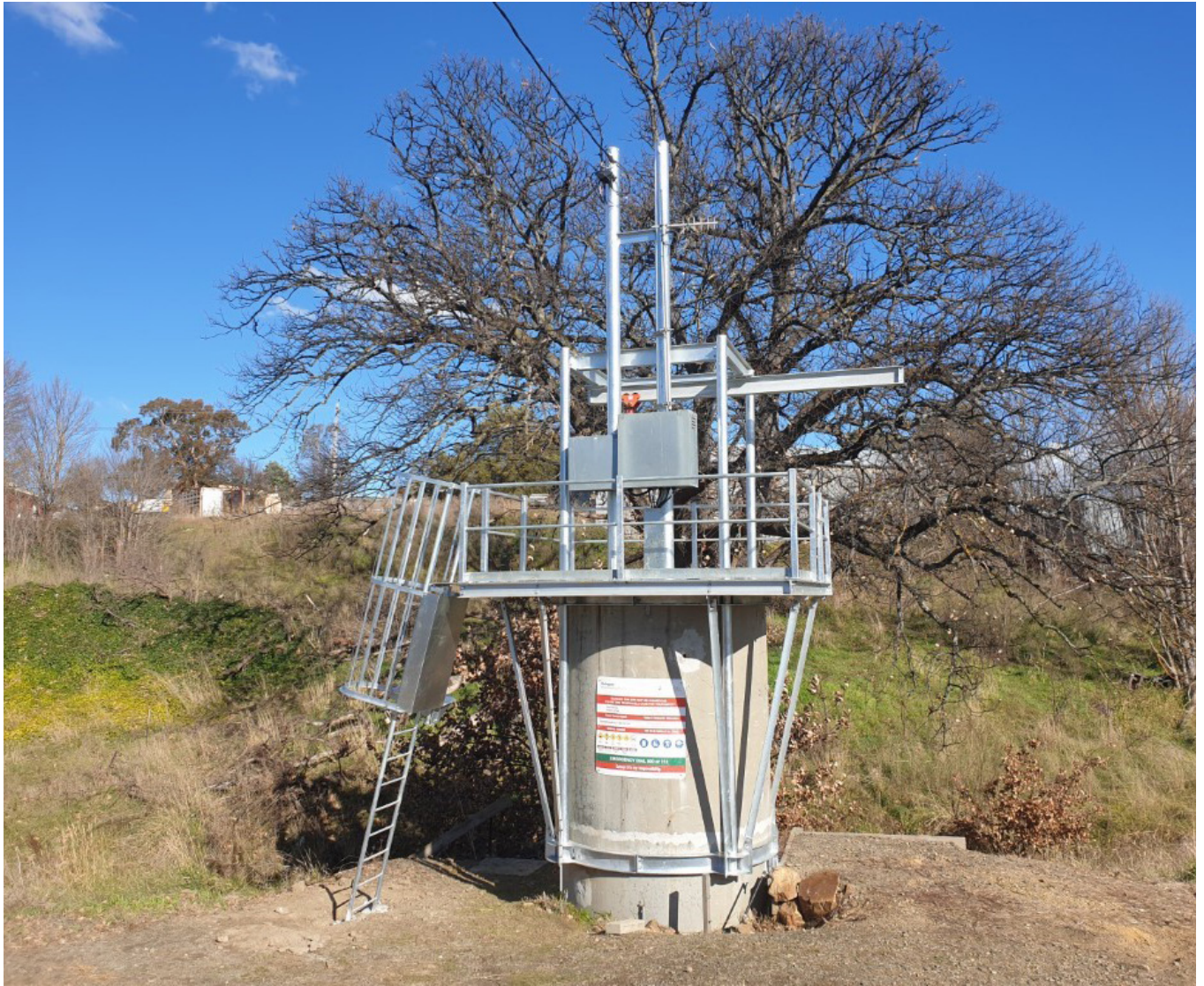
Figure 1: New platform for Delegate Sewage Pump Station
