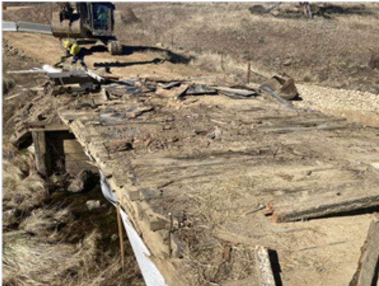
Above: Scotts Creek Bridge (Old Bombala Road)
