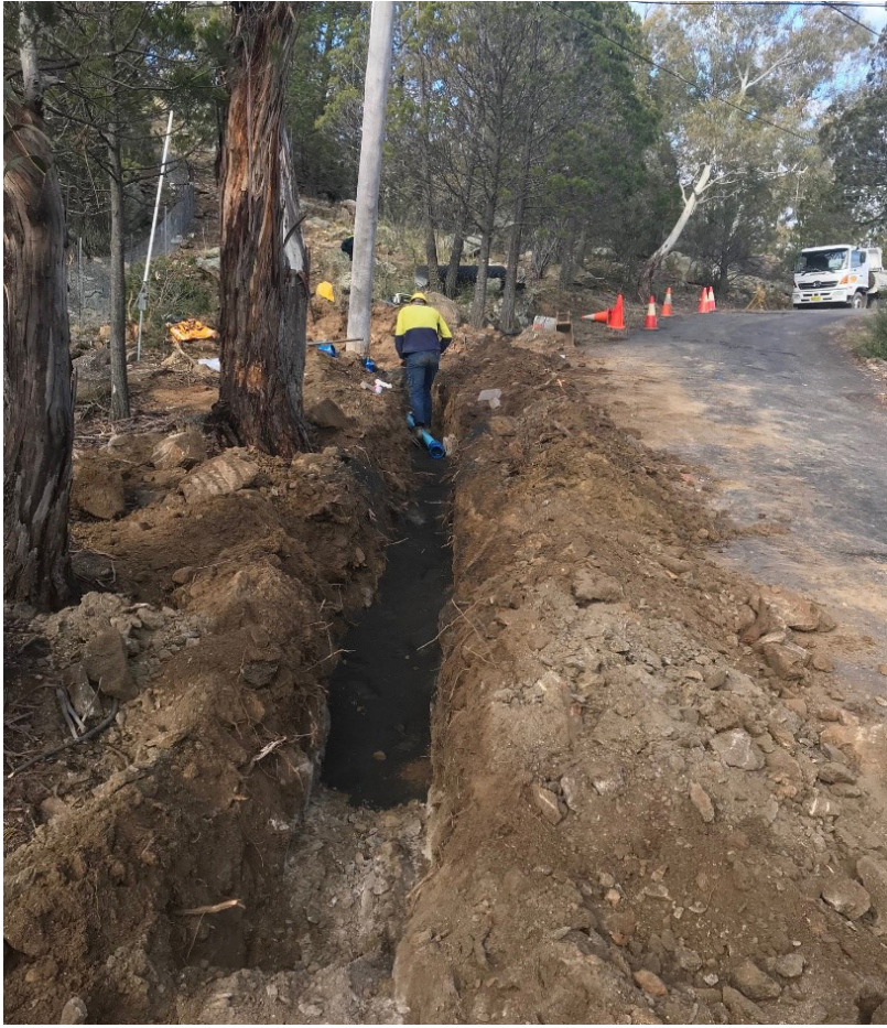
Figure 3: The water team working hard to construct the East Street water main extension in Cooma
