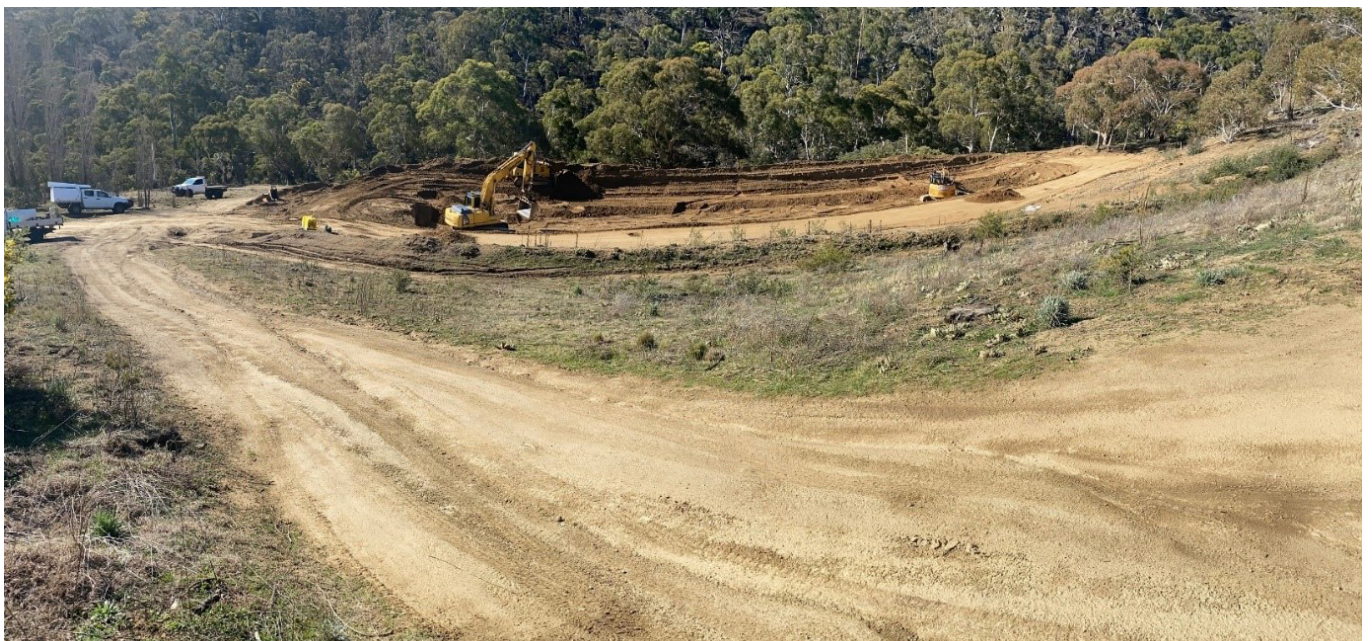
Figure 2: Construction work making good progress on the upgraded evaporation pond at Kalkite Sewage Treatment Plant
