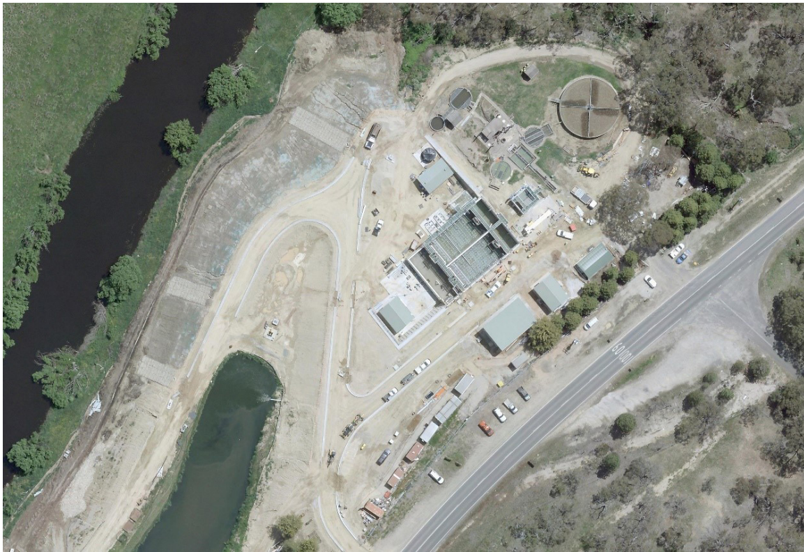
Figure 4: Construction work at Bombala STP in February 2021
