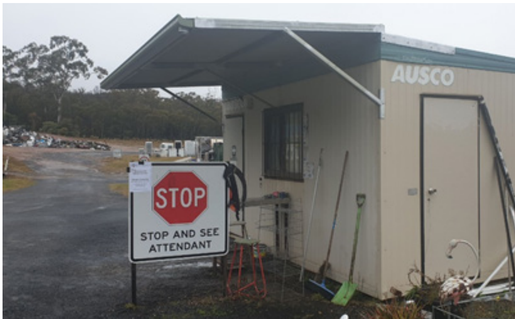
Above: New weather awning for Bombala Landfill site office
