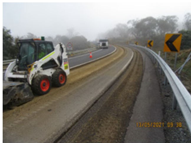
Right: Works being completed on Kosciuszko Road
