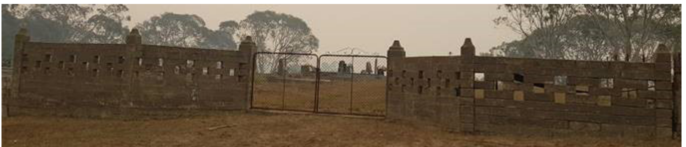
Stone entry wall at Cathcart Cemetery after repairs
