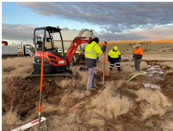
Broken water main, Cooma
