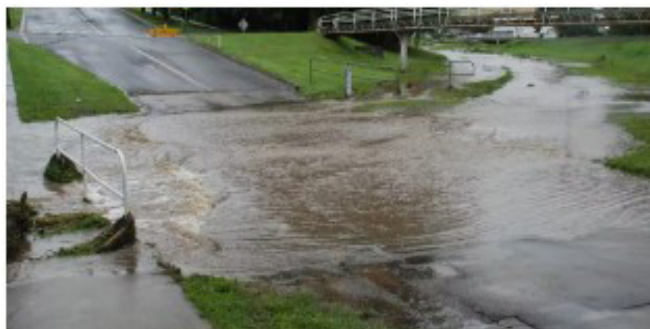
Flooding in Cooma
