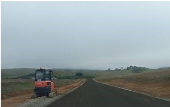
Completed works on Tinderry Road
