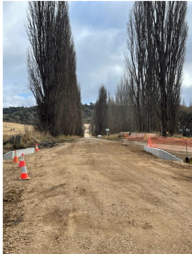
Works undertaken on Michelago Road
