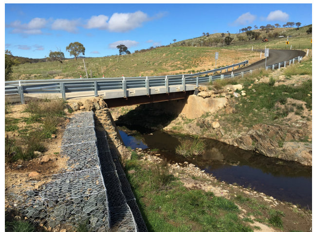
Burra Road bridge works
