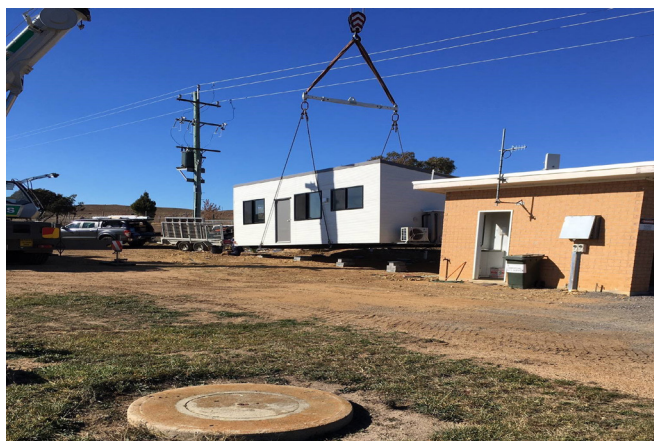
The new lab and office for Delegate arrive onsite
