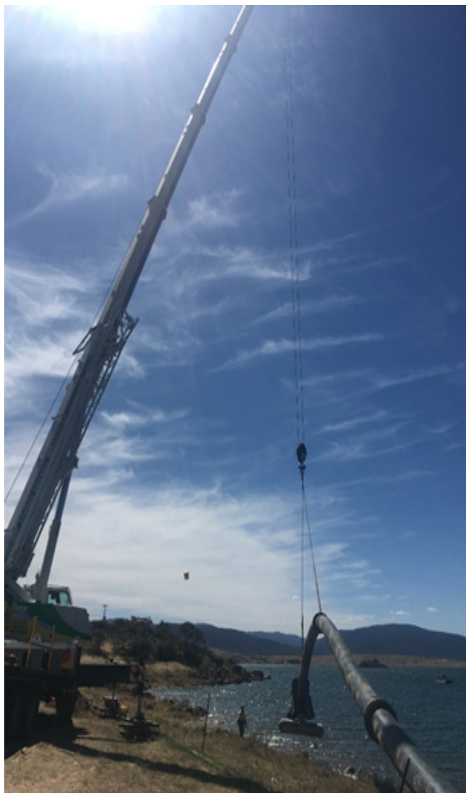
East Jindabyne Water Intake trunnion replacement
