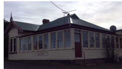
Nimmitabel Community Hall recieved a new roof.
