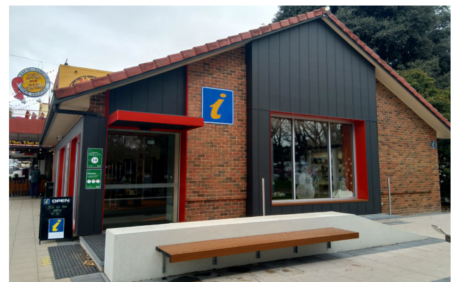
Completed upgrade of the Cooma Visitors Centre
