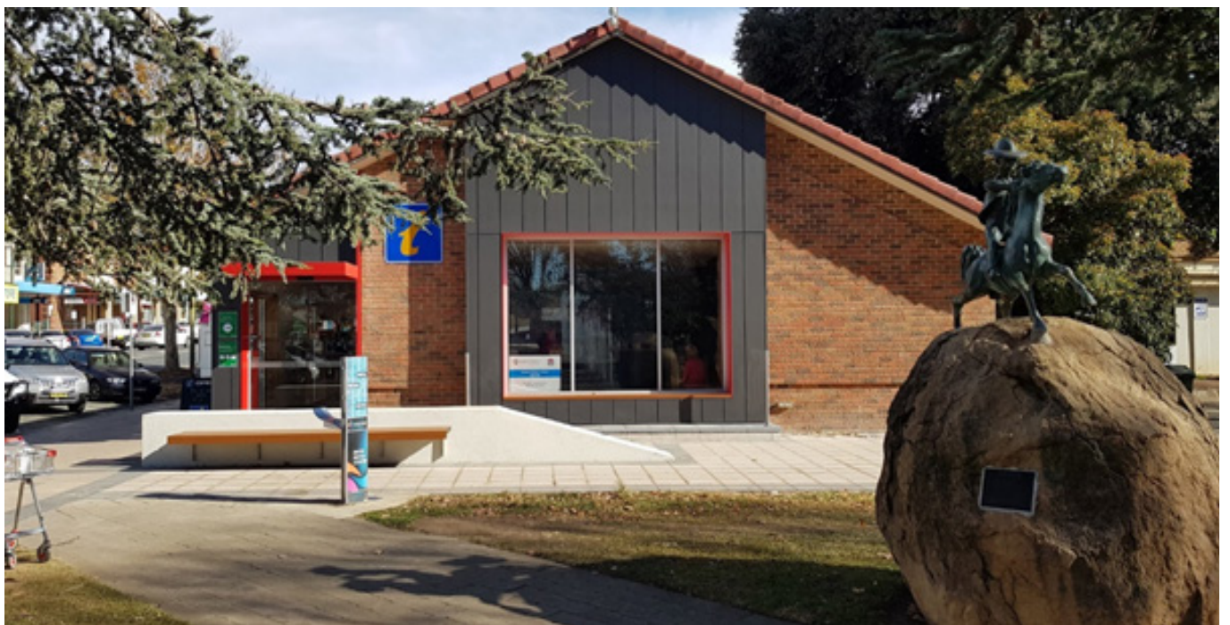
Cooma Visitors Centre upgrade – With Cooma and the Snowy Mountains area becoming a year round travel destination the upgrade to the Cooma Visitors Centre now provides visitors and locals alike with a welcoming information hub to all that the Snowy Monaro area has to offer.
