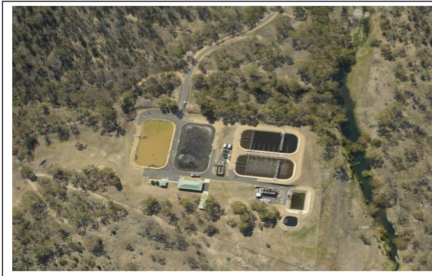
COOMA WASTEWATER TREATMENT PLANT (THE GLEN)
