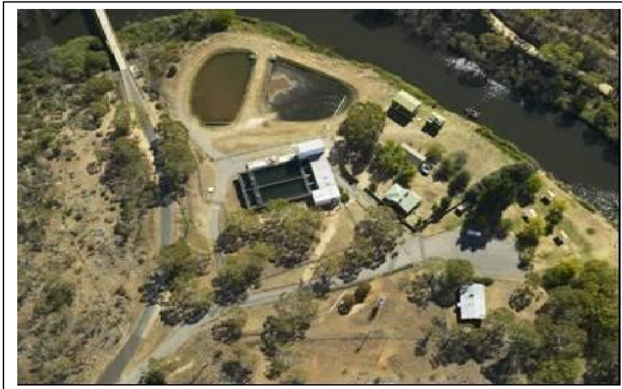
COOMA WATER TREATMENT PLANT ON MITTAGANG ROAD
