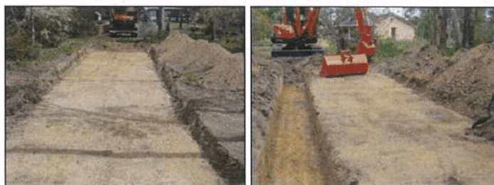
Figure 10.13 and 10.14 Excavation of the bed of the "Wick" trench
