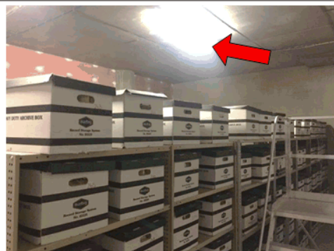
No smoke detection provided in basement archive storage rooms or Floor 2 units
