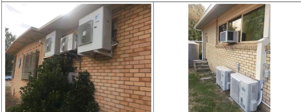
Berridale – Typical split system air conditioning units
