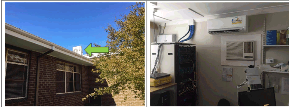
Bombala – Roof mounted split system air conditioning unit and dual units for server room.
