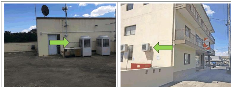
Cooma – Main air-conditioning units for floor 2 on the roof and typical split systems for the offices.
