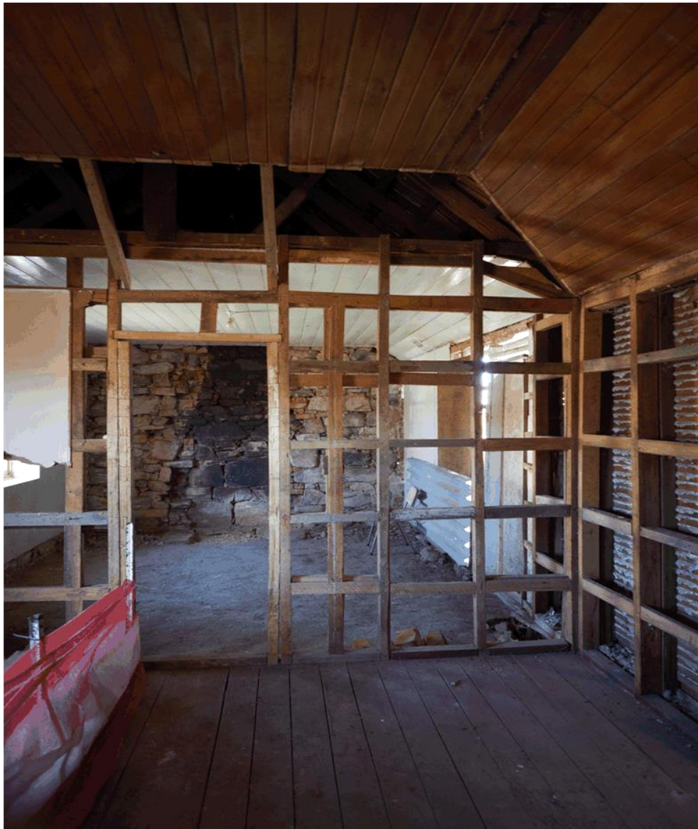
Figure 7: Interior of Aitchison Cottage, showing wall to be removed, August 2017; timber shingles are located above ceiling; photograph: Paul Wallace
