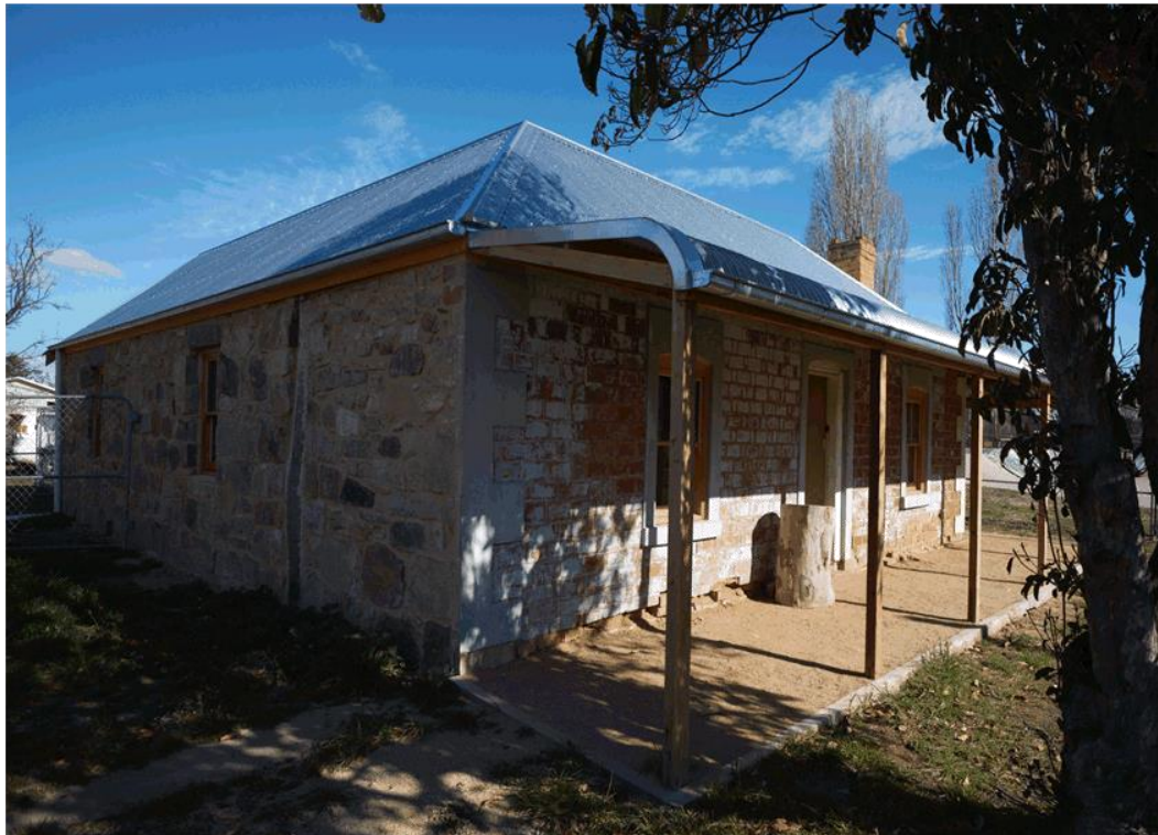
Figure 11: Aitchison Cottage, showing new galvanised iron roof and verandah, rubble stone wall with pole frame at left, and red brick front; photograph: Paul Wallace
