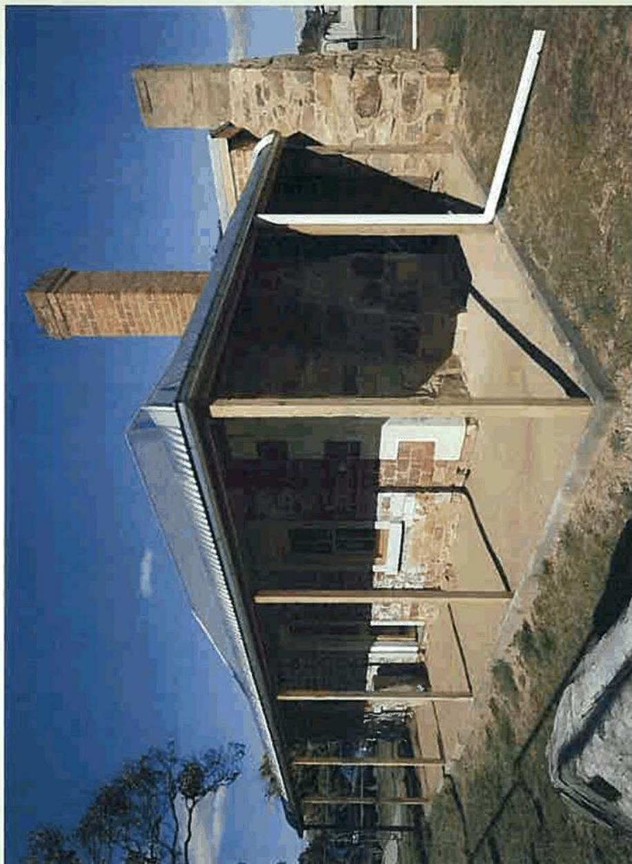
Aitchison Cottage, August, 2017 Restored front and chimney; reconstructed roof and veranda; photograph: Paul Wallace
