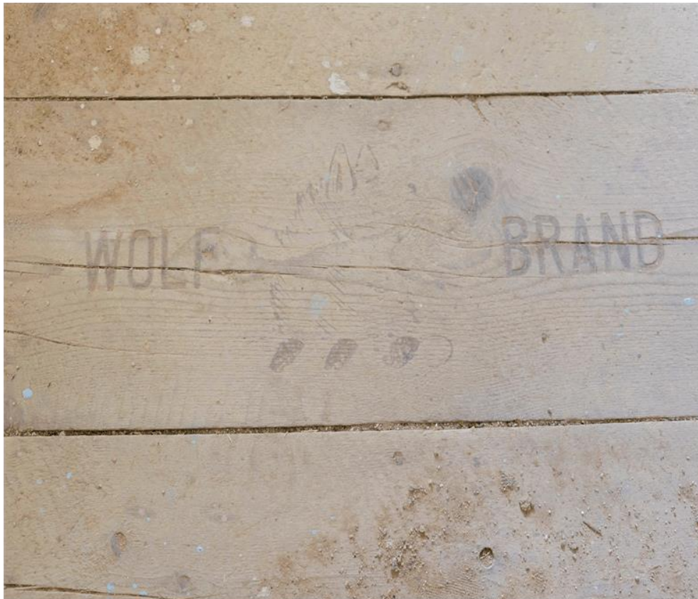
Figure 9: Interior of Aitchison Cottage, showing packing case timber floor boards, August 2017; photograph: Caroline Cosgrove
