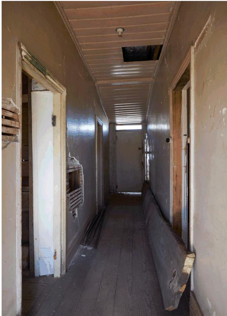
Figure 8: Interior of Aitchison Cottage; hallway showing damaged lathe-and plaster wall on left, August 2017; photograph: Paul Wallace
