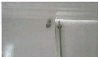
Exit door with barrel bolt from community hall to side path.
