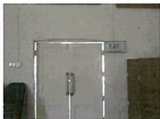
Exit door with barrel bolt from community hall to side path.
