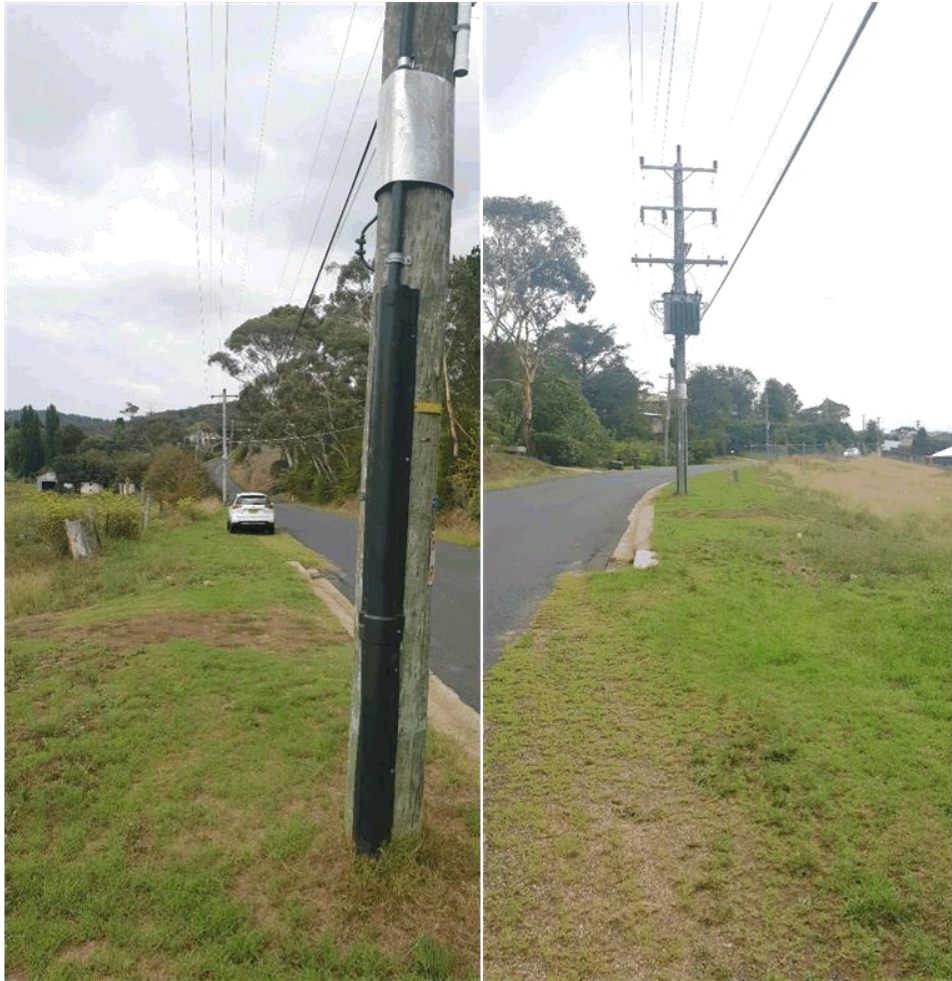
Photos showing overhead Telstra cable at proposed entrance on Hawkins St. Note a join exists at the pole with the transformer. This is not an appropriate location for a join and will need to be relocated.
