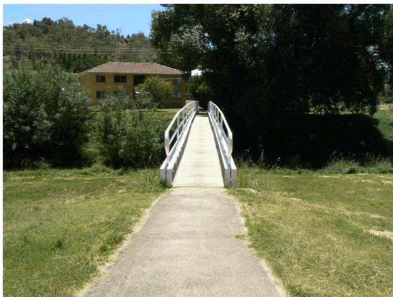
Barrack St - Narrow bridge for pedestrians and bikes over Cooma Back Creek – Wider bridge required
