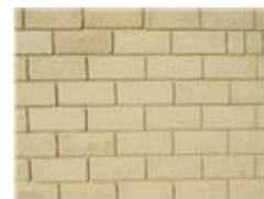
Ground Floor Cladding
