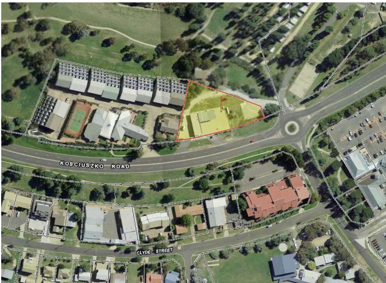
Figure 2 - Aerial view of the site in context with the surrounding land uses.
