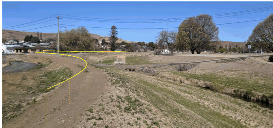
Visualisation of levee raised by approximately 1 m (yellow lines) near Commissioner Street. The average raised amount is 0.4 m but some sections will be around 1 m higher.
