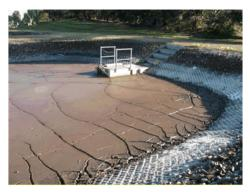
Figure 5 0.6 ML/d Balmoral DAFF main building (left) & Lined sludge drying bed for 23 MLD Hamilton WTP (right)
