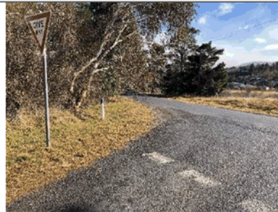
Obscured sight distance
