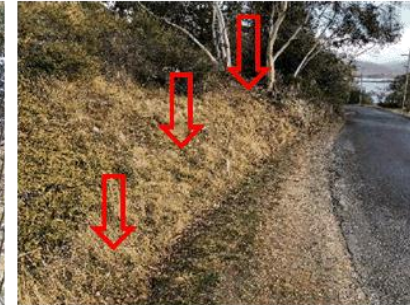
Existing Kanangra Crescent linkage looking uphill from Jerrara Avenue.
