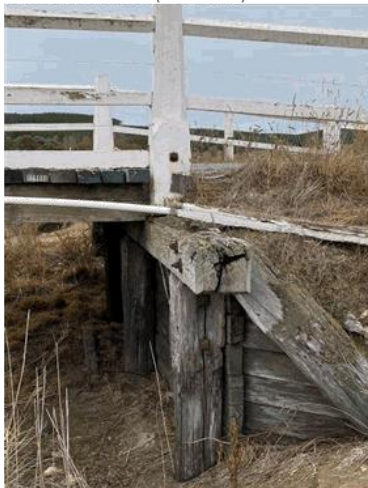
East abutment log split and degraded
