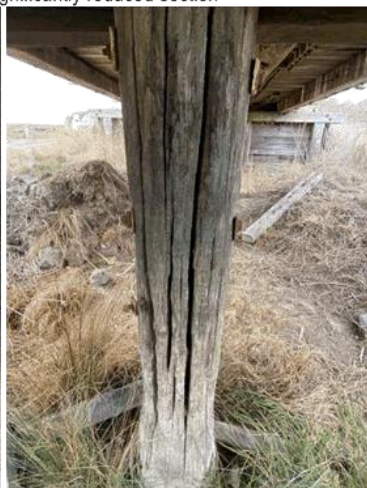
Split,cracked central pile at east headstock
