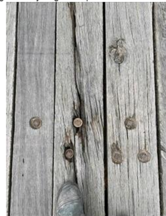
Deck plank degraded
