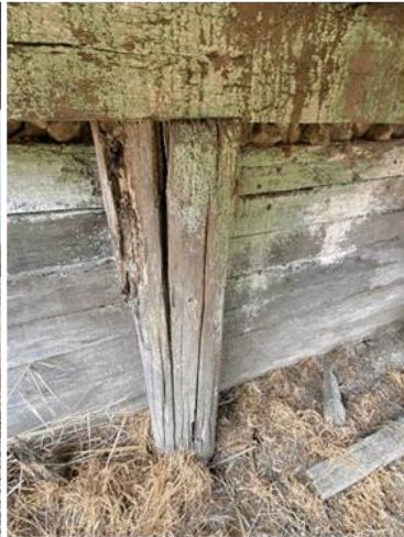
badly degraded east abutment pile
