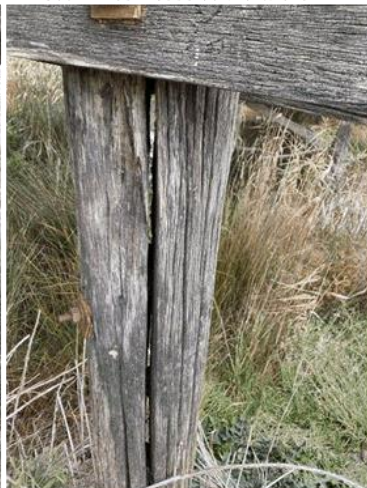
East headstock central split/degraded and significantly reduced section
