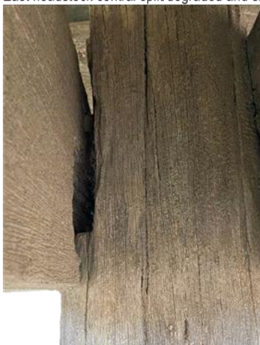
South east pile and headstock separation
