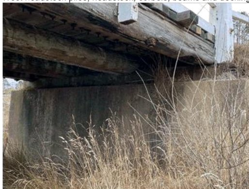
West side concrete abutment
