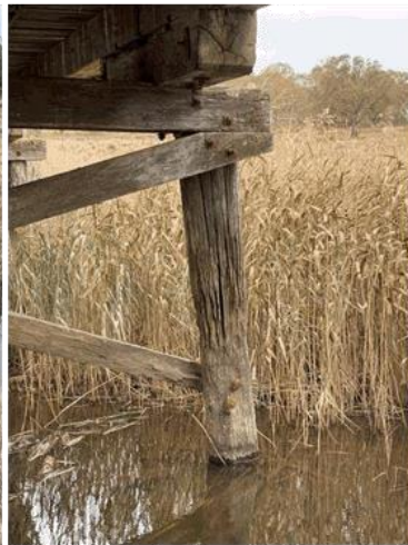
Worn reduced pile at headstock on south west side depicts reduced section
