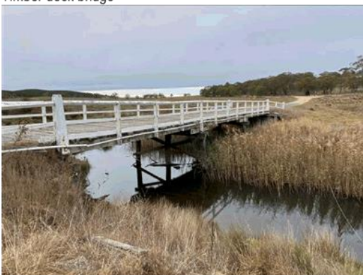
Bridge spans over river
