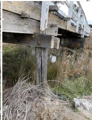
North East (downstream) headstock split
