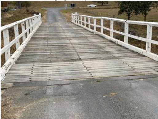
Timber deck bridge
