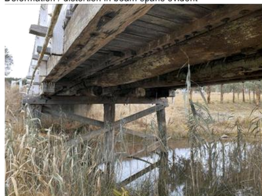
Under deck view from south east side (upstream)
