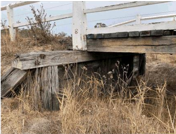
Degraded eastern abutment
