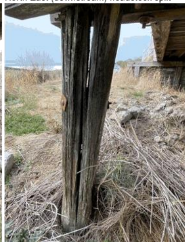
damaged ineffective downstream north pile
