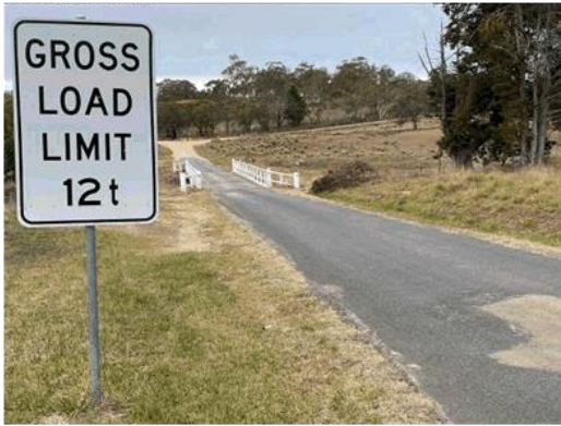
Current Load limits signage to approaches
