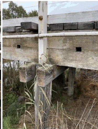
South East headstock (no bracing)
