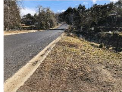
Shoulder constriction at existing culvert (looking north)
