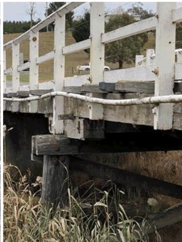
South West headstock/kerb/rails
