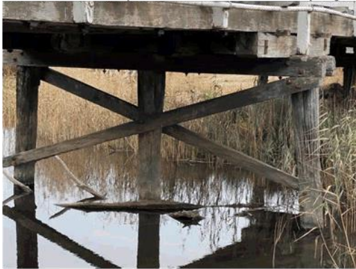
Braced west abutment
