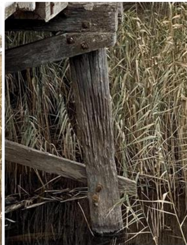
Worn reduced pile at headstock on south west side depicts reduced section
