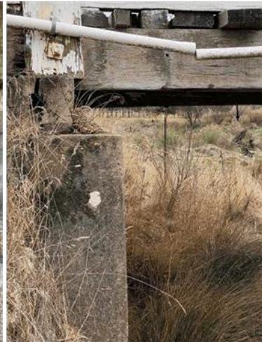
West abutment concrete and beam
