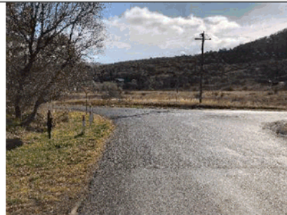
Faded line marking and obscured Give Way sign
