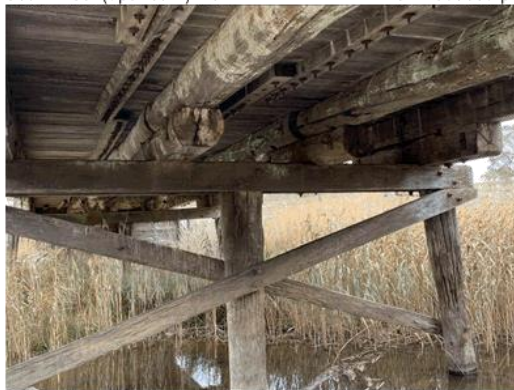
West headstock piles, headstock, corbels, beams and decking
