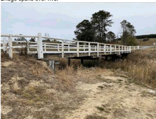
View from north east approach
