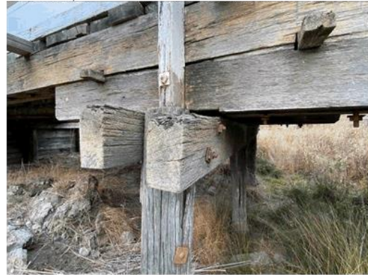
South east headstock (downstream) ineffective beam displaced and parted from significantly degraded pile
