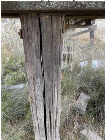
East headstock central split/degraded and significantly reduced section
