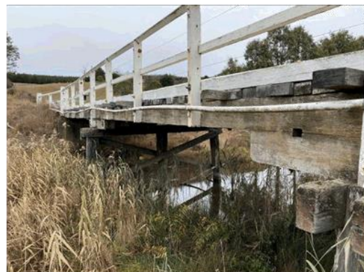
Deformation / distortion in beam spans evident
