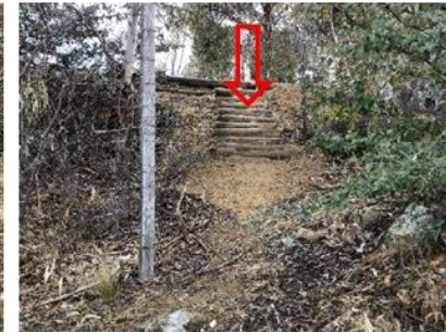
Existing Camira Avenue linkage looking uphill from just below Camira Avenue
