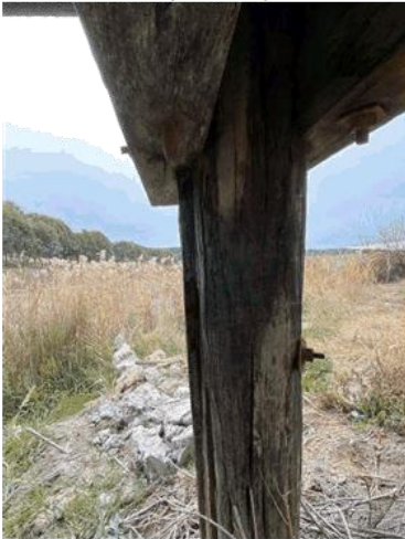
North east headstock pile ineffective
