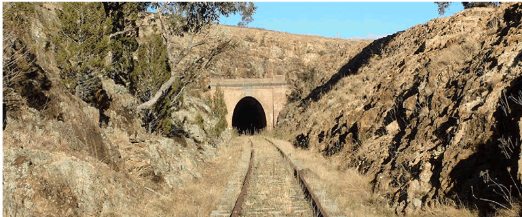
The Colinton Tunnel is one of the unique features of this disused railway line and will be a major attraction to users if the trail is developed.
