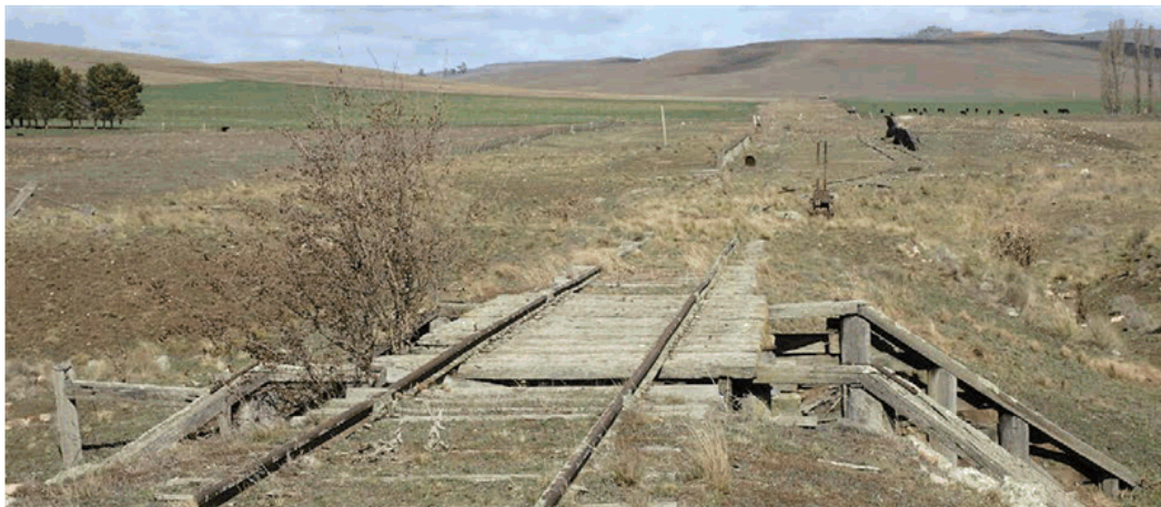
Elements of the remaining infrastructure include bridges, sidings, switches and, in some locations, the original stations, signals and distance pegs.
