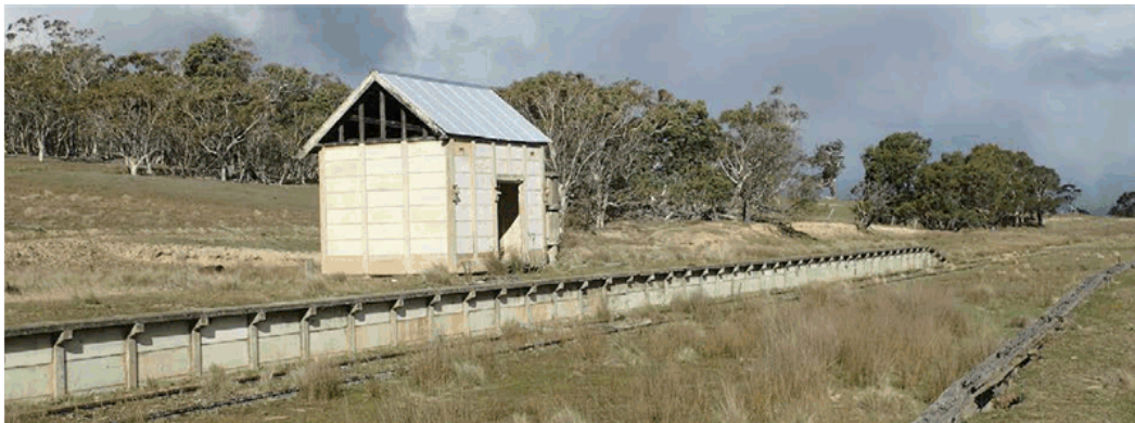
The old siding building at Bukalong would be the destination for pedal cars, should the plans of the Friends of Bombala Railway Inc. ever come to fruition. The building would need renovation if a rail trail was to be developed (and could be useful as a toilet and/shelter).
