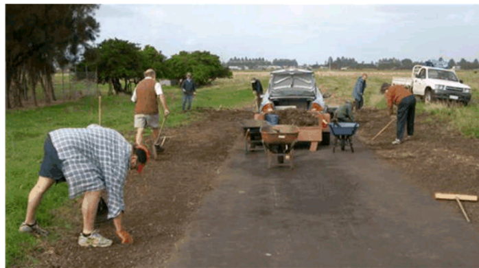
Volunteers organised by the Committee of Management at a busy bee to undertake maintenance work along the rail trail near Port Fairy in western Victoria.
