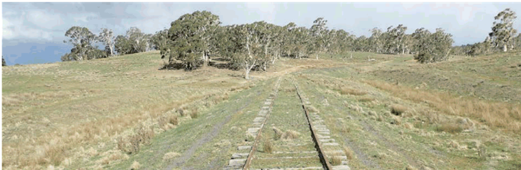
A typical scene along the corridor south of Cooma (north of Bukalong siding). The railway south of Cooma was developed without fencing and without ballast.
