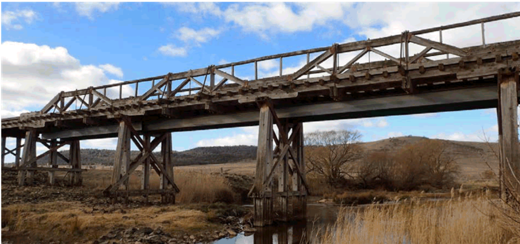
Although in poor condition, the 390m bridge over the Numeralla River is spectacular and would be a major attraction along the proposed rail trail.
