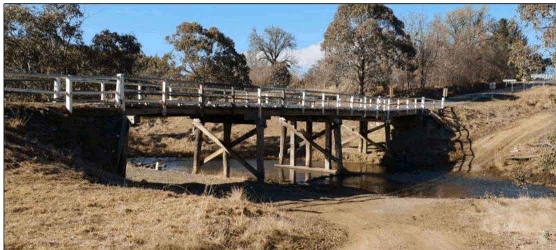
Figure 2-13: Side view of the bridge looking towards Abutment 2 end of the structure. Note the dip in the bridge at Pile Bent 3 on the opposite bank of the river. Pile Bent 3 has settled over time or was installed incorrectly.
