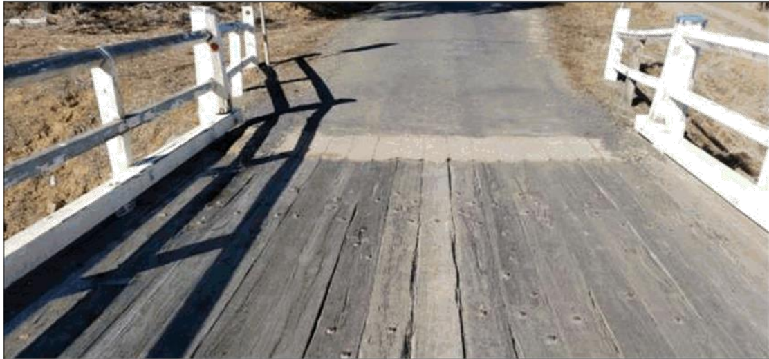
Figure 2-25: View of approach at Abutment 2 showing the condition of the asphalt approach is fair condition with no signs of abutment fill settlement.
