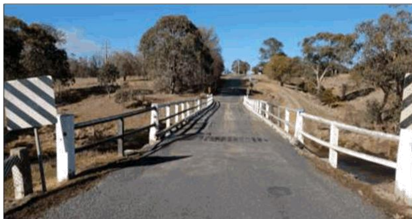
Figure 2-28: The timber and metal rails fan away from the bridge on both sides of the bridge to help guide traffic on approach to the structure.
