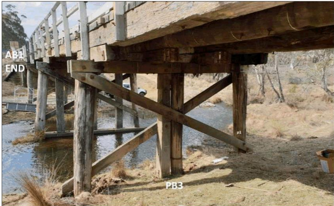
Figure 2-14: View of Pile Bent 3. Pile 2 has an extra pile installed next to which is bearing on a concrete footing. Pile 4 has visible deterioration just below the ground line. Also, water flowed out of the shallow inspection hole dug around Pile 4 during the inspection indicating the ground water table is higher than the current stream elevation.
