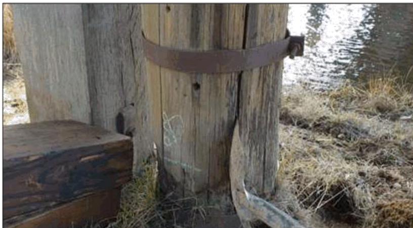
Figure 2-18: Several piles have vertical splits through the length of the member. Moisture can enter into these areas and start to decay the heartwood. Also, many of the piles have steel compression bands which were installed in an attempt to keep the piles from expanding and splitting. The use of metal banding is a poor practice and typically does nothing to stop the natural process of timber shrinkage and expansion and buckling inward of the pile.
