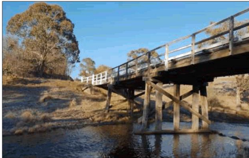
Figure 2-6: View of Delegate River Bridge looking north. The bridge is comprised of four spans consisting of three timber pile bents and two timber abutments with planked back walls. Each deck span is supported with log girders that rest on timber corbels on top of timber headstocks.
