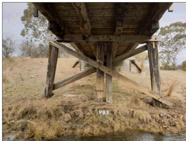
Figure 2-21: View of Pile Bent 3 looking south. Bent 3 consists of four piles and two cross braces with some visible decay at the lower parts of the piles.
