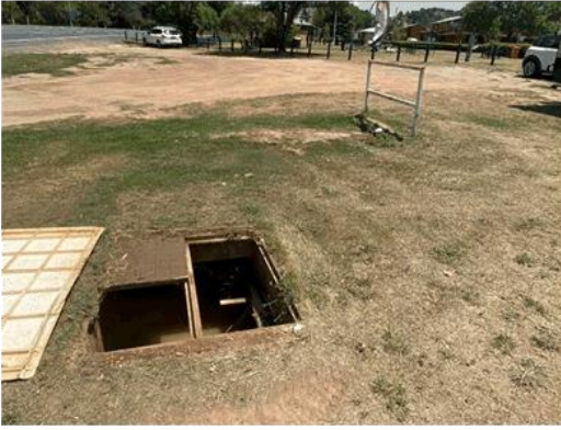
Existing Telstra pit and inappropriate lid (will need a proper lid for the proposed truck stop)
