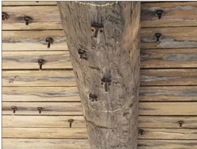
Figure 2-12: View of the vertical through bolts which hold down the deck planks. Note the difference in colour around each bolt where moisture has been present. These areas will begin to decay over time. Vertical bolts that penetrate from the top surface allow moisture a direct path to untreated heartwood and accelerate the decay process.
