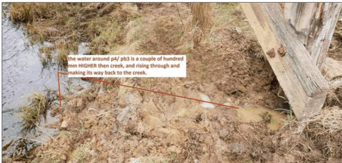
Figure 2-15: Close up view of Pile 4 in Pile Bent 3 showing the water flowing out of the inspection hole.
