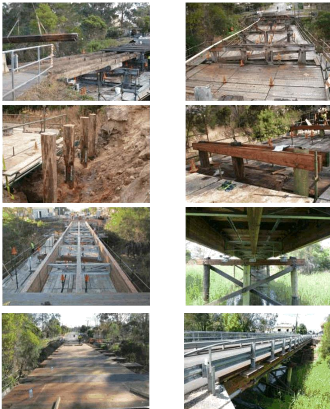
Figure 5-5: Replacement of Bob Wells Bridge in Cessnock, NSW. The original superstructure and deck were removed, the substructure was restored utilizing high strength fibre wraps on the timber piles, and prefabricated Penta-treated glulam girders and deck were installed. The completed system has a life expectancy of 75-100 years.
