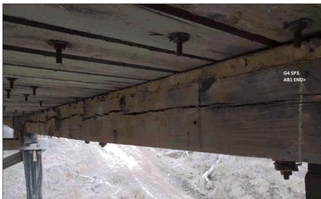
Figure 2-17: Girder 4 in Span 3 was found to have a horizontal crack along the entire length of the member parallel to the grain. Moisture can enter into these areas and form pockets of decay inside the member weakening its structural capacity. Girder 1 in Span 3 is in a condition similar to Girder 4.
