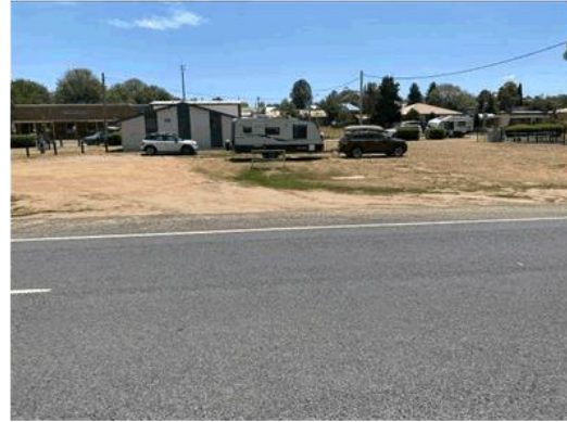
Existing toilet and gravelled parking area
