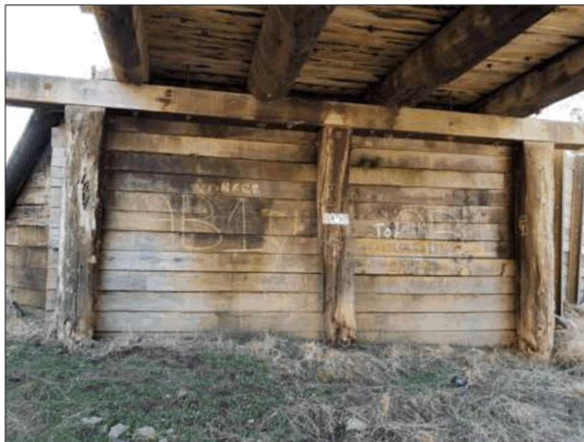
Figure 2-7: View of Abutment 1. The timber back wall planks are in a fair condition, with little to no gaps between the individual planks. When back wall planks are nailed to the piles this can often cause problems as the shrinkage and expansion of the timber over time creates gaps between the planks, allowing the erosion of fine sediments from the approaches. Also note the splits and the decayed areas of the piles near the ground.
