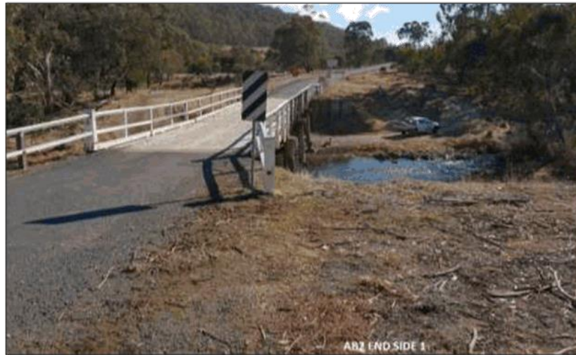
Figure 2-2: View of bridge from Approach 2 travelling towards Bombala. This approach is also asphalt, the same as Approach 1.
