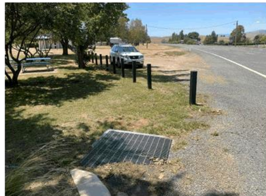
Closer view of existing drainage pit to west approach to park
