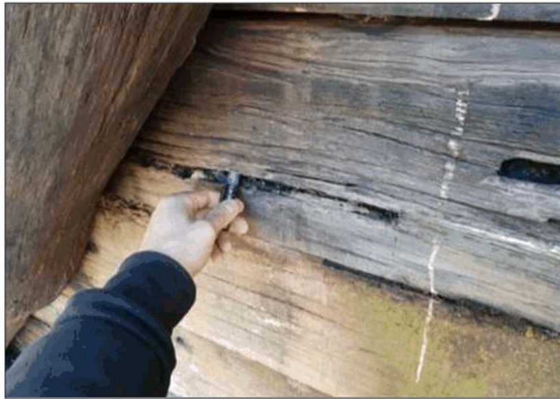
Figure 2-8: Both abutments have timber wing walls on both sides. Significant decayed areas were found in the wing wall planks of the abutments. As seen above, these areas are 25-100mm deep allowing a pen to be fully inserted into the cavity. The structural integrity of the planks at these locations has been compromised.
