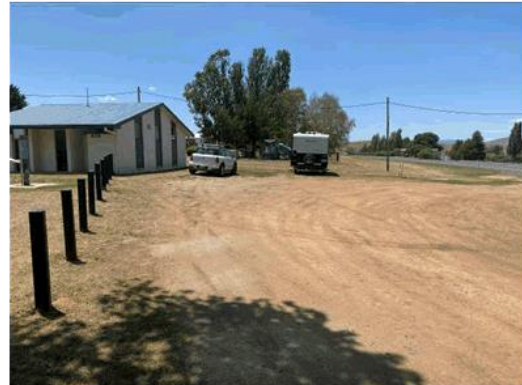
bollards towards the existing toilet
