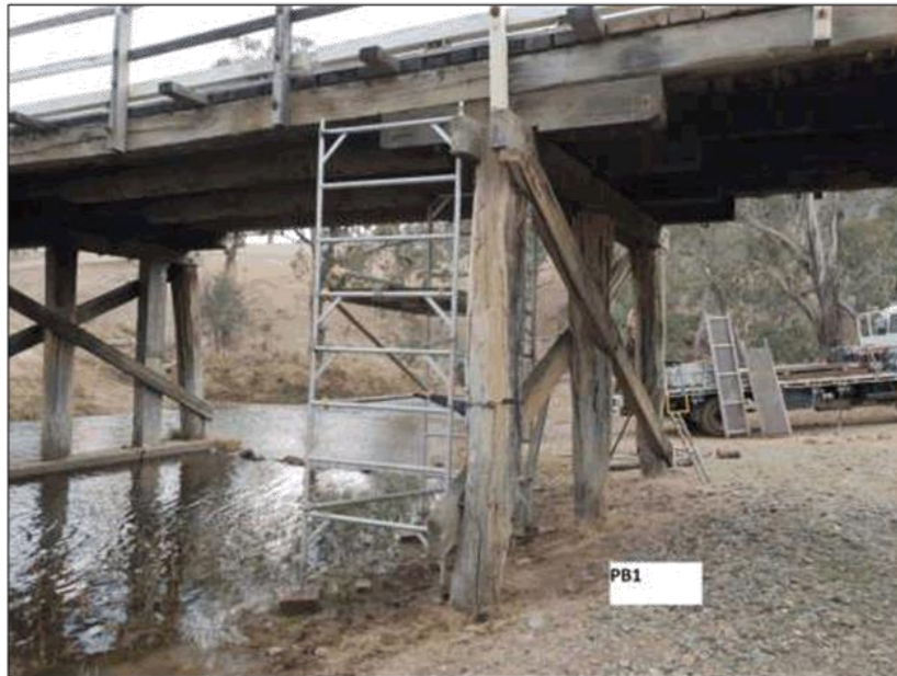
Figure 2-10: The corbels at Pile Bent 1 are in fair condition with little to no exterior decay. The corbels are used to increase the bearing seat area for the girders. Contrary to popular opinion they do not shorten the girder span.
