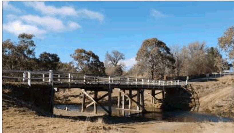
Figure 2-27: The structure was found to be free of any debris build-up.
