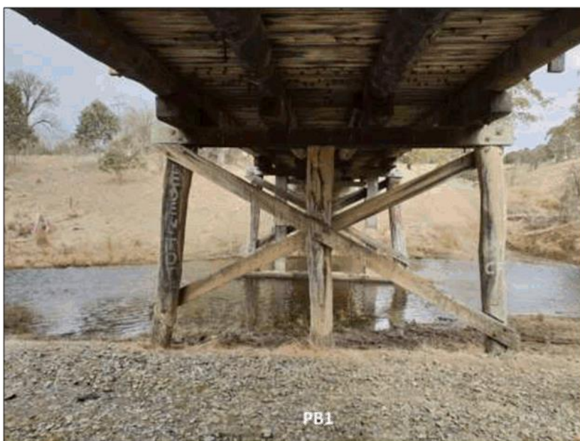
Figure 2-19: View of Pile Bent 1 looking towards Abutment 2. The bent consists of three piles and two cross braces. All three piles visually appear to be in a fair condition, with the exception of the compression cracking that has occurred on Pile 2, due to an inaccurate connection detail of the headstock to the post. All three intermediate bents have this inaccurate connection detail. See Section 2.1.2, after the pictures in this section, which discusses proper split headstock connection details. This bent should have a wale installed.
