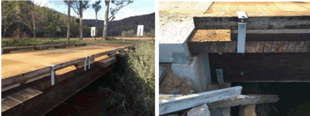
Figure 5-2: Kerb repairs completed for Cessnock City Council on Dairy Arm Bridge included installation of hold downs that wrap around the kerb, and connect to the underside of the deck. Eliminating connections through the top of the deck prolongs the life of both the deck and the kerb.
