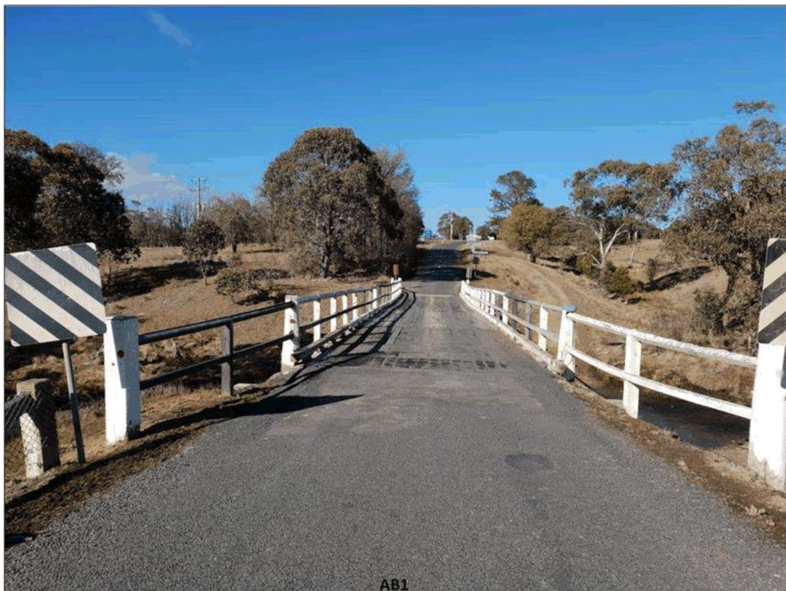
Figure 2-1: View of the bridge from Approach 1 travelling away from Bombala along Delegate Road. The asphalt approach surface allows for a smooth transition onto the bridge for vehicles. The timber and metal guiderail system extends off the bridge at both ends to help guide the approaching traffic onto the single lane bridge. The rail system and kerb have been painted with a heavy solids paint (over 29%) which should be removed and a stain applied to create the same appearance but will not seal in the moisture and promote decay in the elements. Vertical fasteners down through the kerb should be removed and over wrap fasteners utilized instead to prevent the promotion of decay within the elements by the access from above by ambient surface water.
