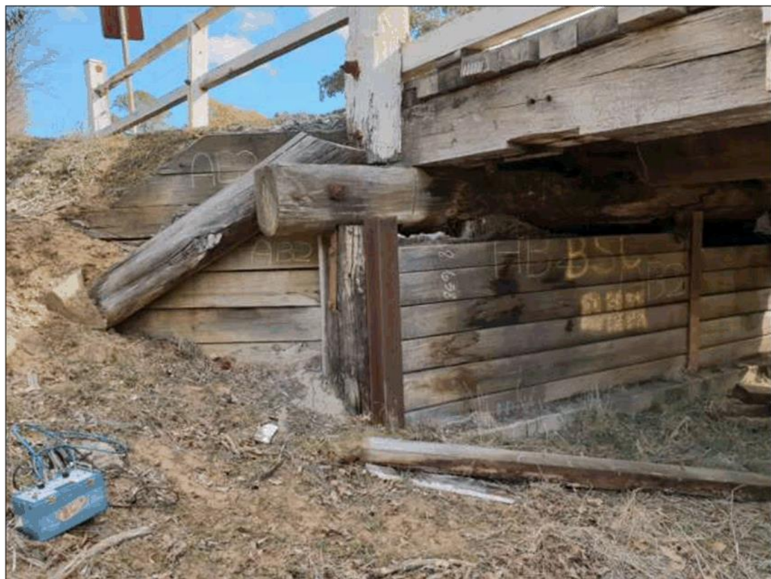
Figure 2-24: Abutment 2 is adequately protected by the timber wing walls and although there is little natural vegetation around the abutments they appear to be stable.
