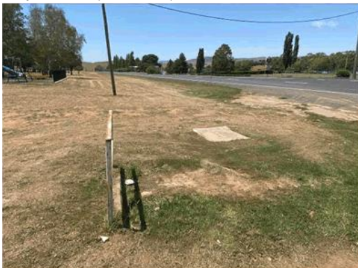
Existing Telstra pits and fence/kerb (purpose unclear)
