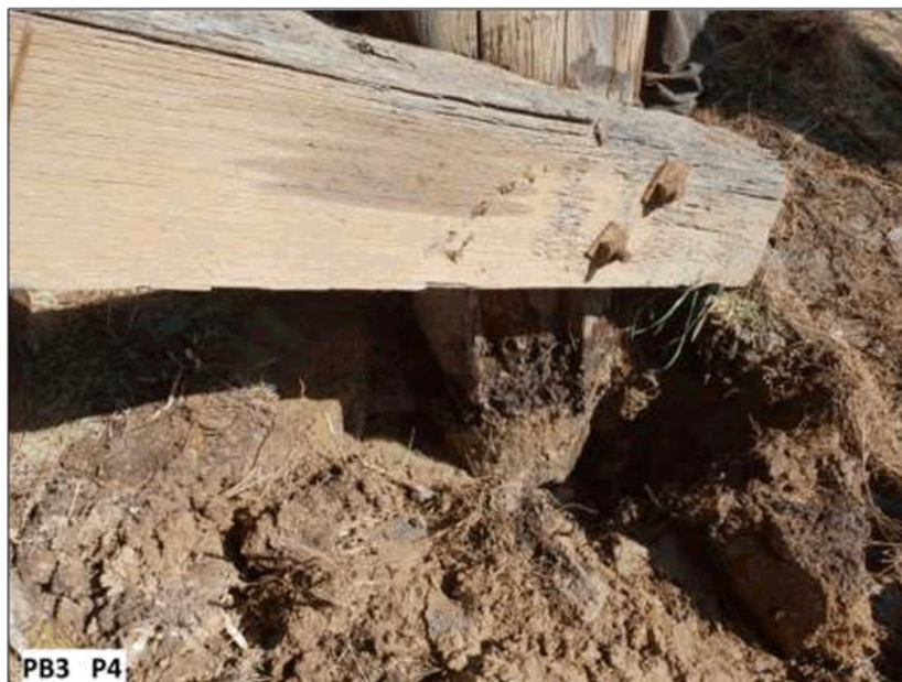
Figure 2-9: Pile 4 at Pile Bent 3 shows signs of significant decay at the ground line. This decay is most likely due to the high levels of moisture in the soil from the elevated water table combined with the presence of oxygen near the soil surface.
