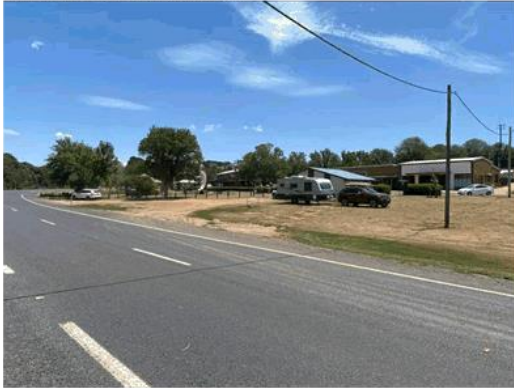
Existing gravelled area showing poles
