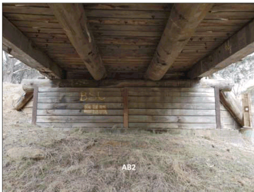
Figure 2-22: View of Abutment 2. Timber back wall planks are in fair condition with some of the girders heavily notched at the abutment seat. Also note the girders are more than a distance of D (depth of the split headstock) away from the pile tops which makes the headstock susceptible to horizontal shear cracking.
