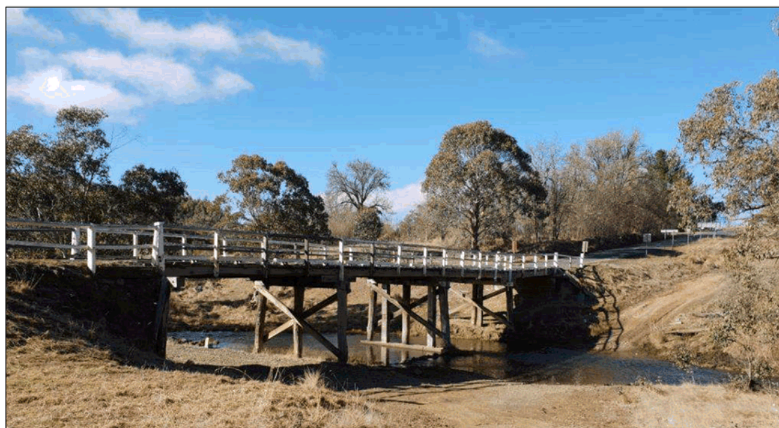
Figure 2-23: Delegate River follows a stable path under Spans 2 and 3 and shows no signs of past or imminent stream migration.
