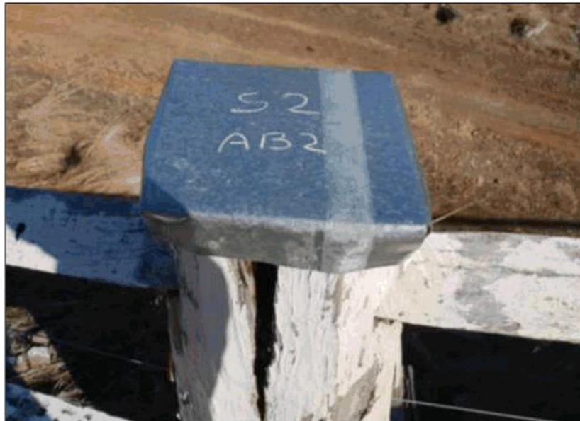
Figure 2-5: The tops of the handrail post have metal caps installed in attempt to prevent decay. The metal caps instead trap moisture and promote decay if not installed properly. The metal caps sweat and condensate water with change in temperature.
