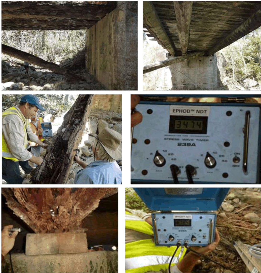
Figure 5-1: Photos showing global failure of a timber log girders. Both failures were caused by advanced decay in the ends of the girders and transverse shear failures. Vertical fasteners were the primary cause of this decay. These failures were found in elements with SWT values in the 3000 \mu s to 6000 \mu s range. Typically, similar bending extreme tensile fibre failures in log girders occur in zones of decay where there are over 2000 \mu s SWT values. Similarly, if vast portions of the log girder have SWT values over 33000 \mu s the failures may occur.
