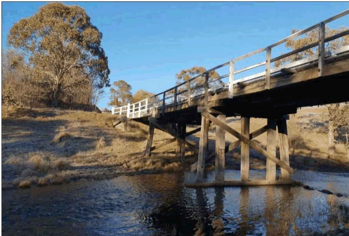
Figure 2-26: Pile Bents 1 and 2 appear to be stable. Pile Bent 3 appears to be stable but is lower than the other bents.
