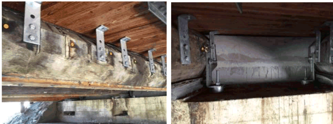
Figure 5-3: A deck replacement on Mars Road in Cassowary Coast necessitated connecting new glulam deck panels to existing girders (Left). The angles used allow for connection to a range of sizes of girder, and eliminate connections through the deck and into the centre of the girder. Additionally, vertical connectors were removed from the ends of the girders, and angles were attached to the concrete abutments that connected to the sides of the girder (Right), again eliminating vertical connections and extending the life of the member.
