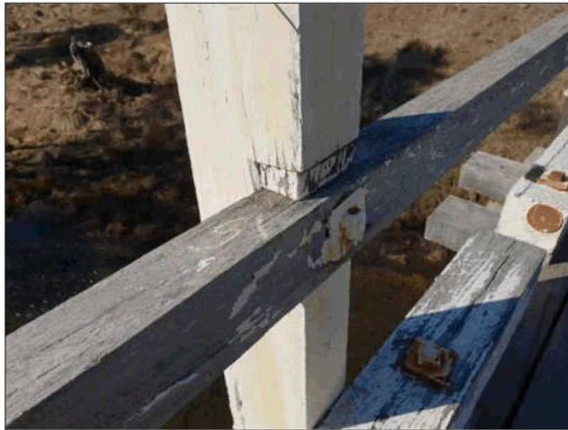
Figure 2-4: The kerb and guiderail on both sides of the structure are in a fair condition even though they have been coated with heavy solids paint. Heavy solids paint accelerates decay by trapping the moisture in the element. A stain with less than 29% solids should be utilized when heavy dimension timber (minimum dimension greater than 50 mm) is to be coated.
