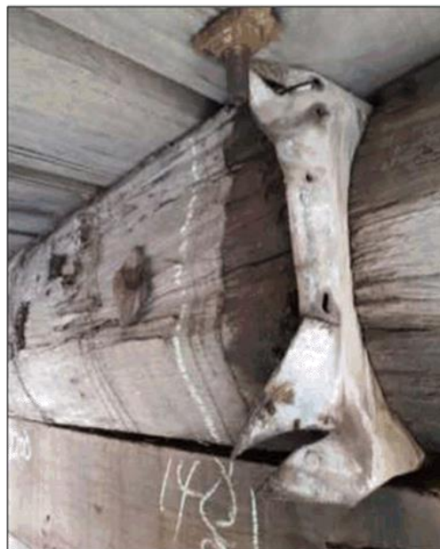
Figure 2-11: At the location where the two girders meet on top of the corbel a metal cap has been installed to cover the ends of the girders. These types of caps prevent water from expelling from the end-grain of the timber. These caps will lead to decay at these locations if not removed and the wood treated.
