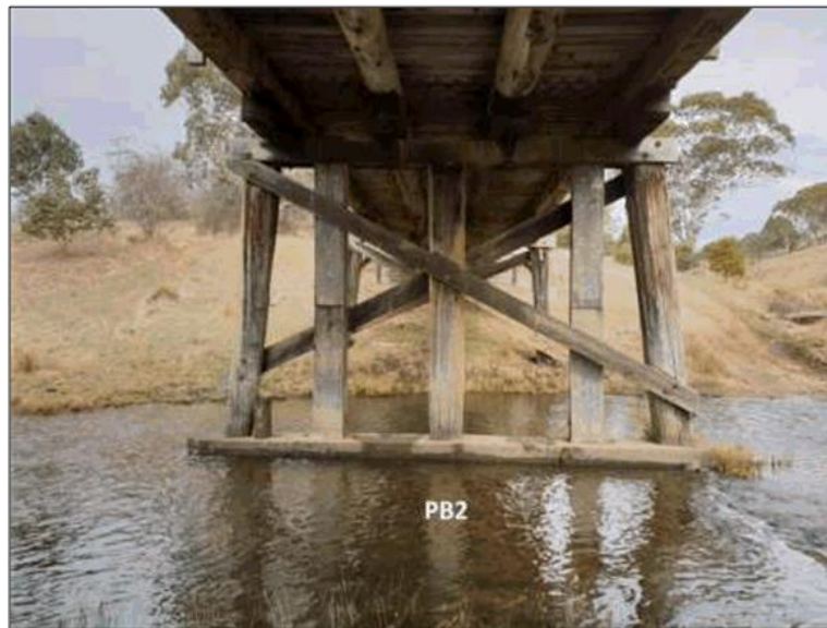
Figure 2-20: View of Pile Bent 2 looking south. This bent consists of five posts and two cross braces resting on top on a concrete sill. Posts 2 and 4 appear to have been posted due to their shape, connection angles and the presence of a malthoid barrier at the concrete sill. The other three posts appear to be encased in the concrete sill. The practice of encasing timber with concrete will lead to the deterioration of the timber within and around the concrete encasement. Concrete encasement holds the moisture content in the wood over 22% MC the point at which wood begins to decay.
