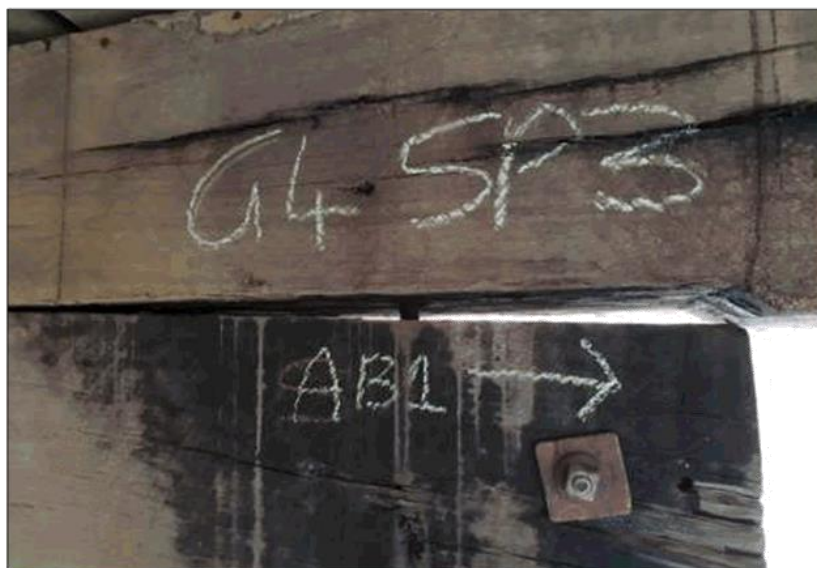
Figure 2-16: Close-up view of Girder 4 in Span 3 over Pile Bent 3. Note the gap between the girder and the corbel which further suggests Pile Bent 3 is now lower than the other bents.
