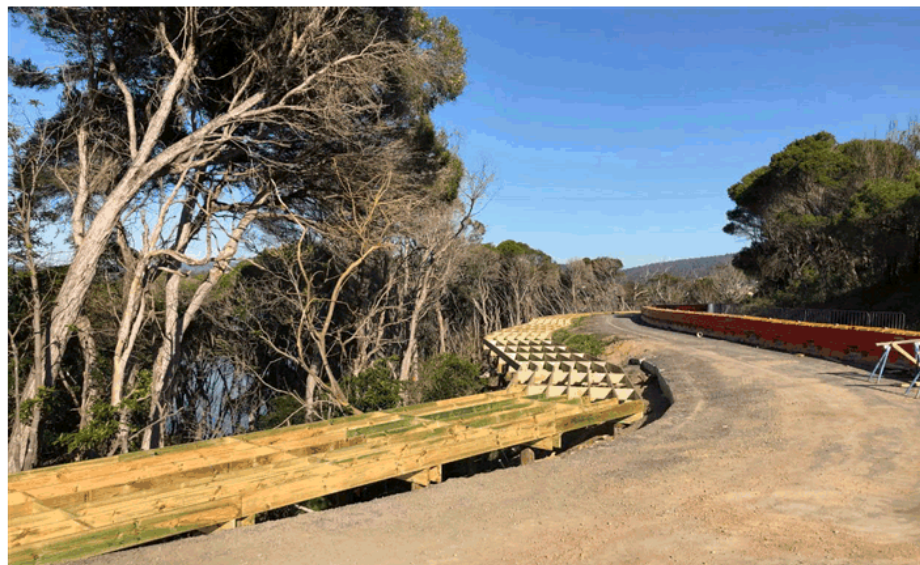
Figure 3-2 Dongwha treated sawn timber used in a pedestrian walkway in Merimbula
