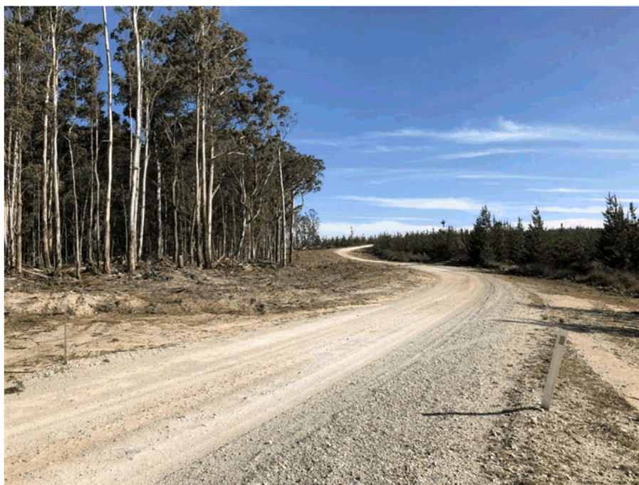
Figure 6-3 Traditional Mineral Earth Firebreak Coolangubra Forest Way
