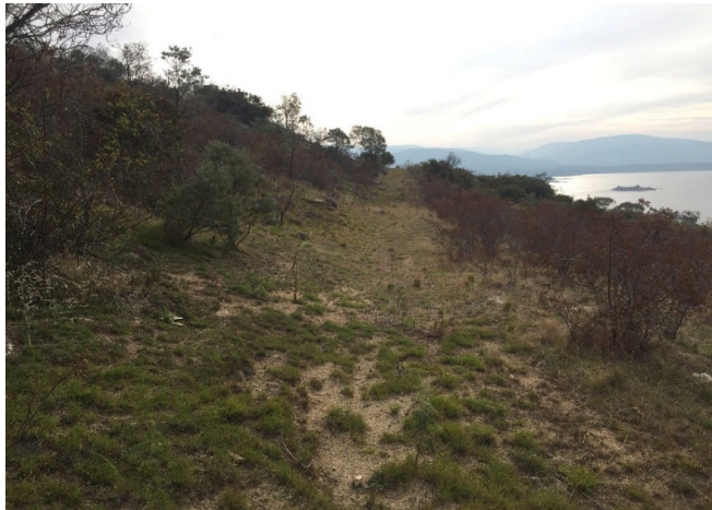
FIGURE 2- EXISTING 4WD DRIVE TRACK- 2 METRE WIDE BENCHED CONTOUR IN PLACE
