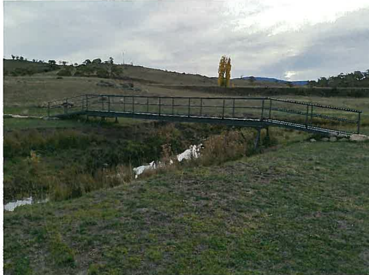
Figure 8 – Wollondibby Creek Bridge on Hatchery Bay Track
