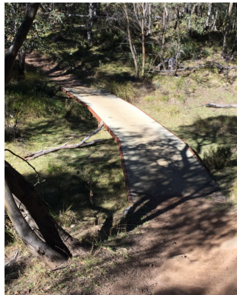
FIGURE 4. PLATFORM EXAMPLE- THREDBO VALLEY TRACK CREEK CROSSING
