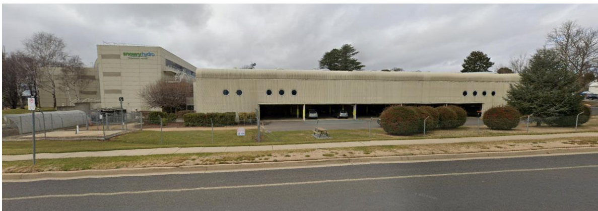
Figure 4 - Snowy Hydro Administration Building to the east of the site.
