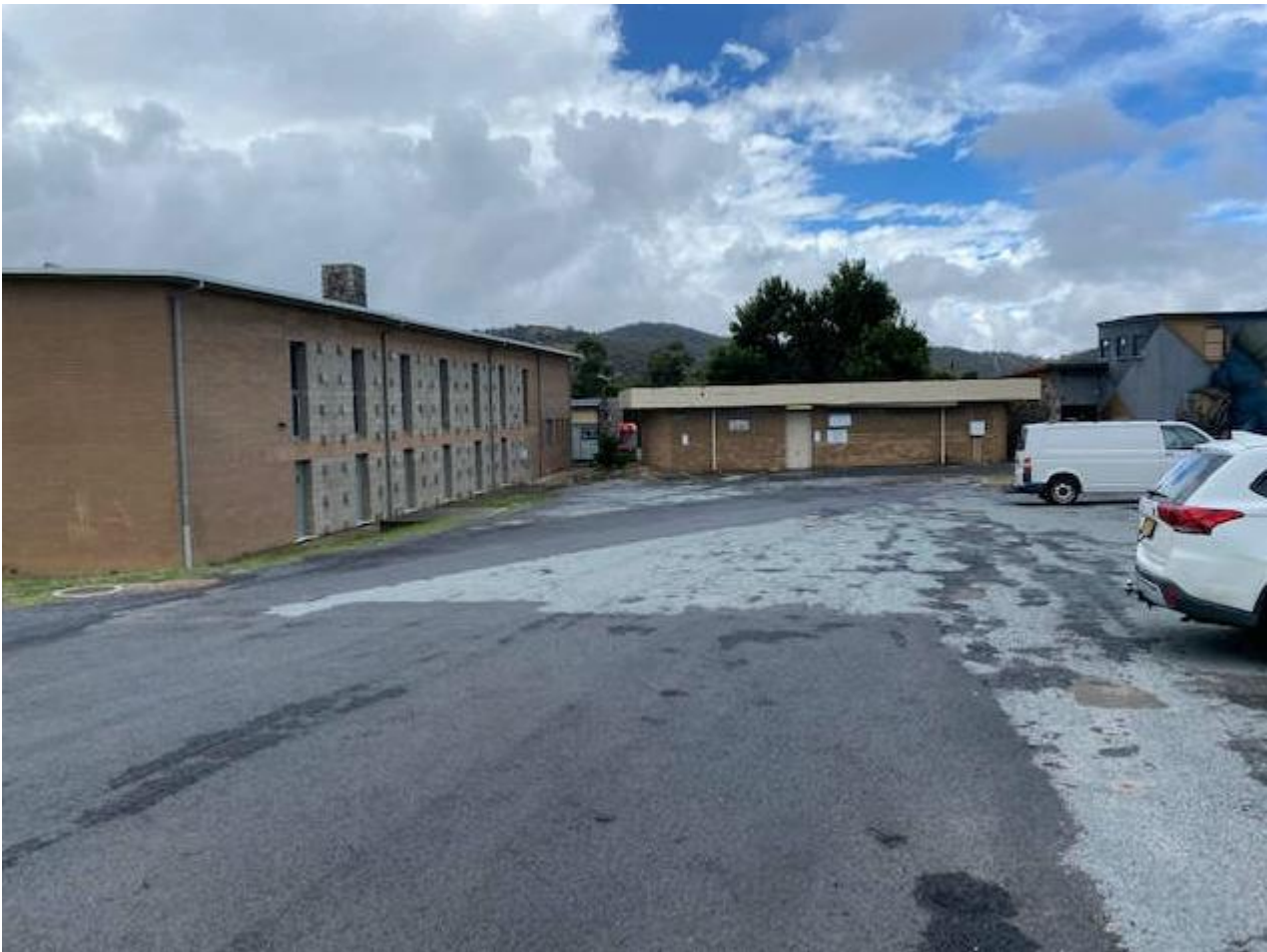
Figure 5 – A view of the adjoining car park showing the rear and side of Jindabyne Memorial Hall and public toilet block
