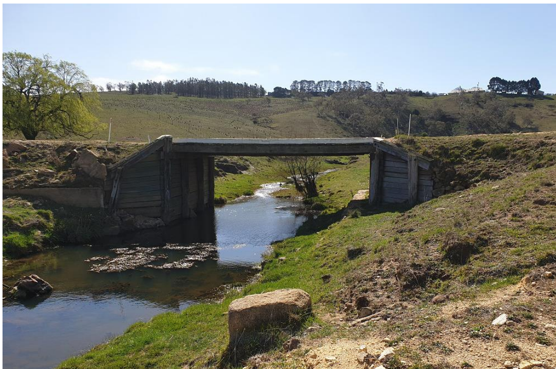
Palerang Bridge, Cambalong Creek
