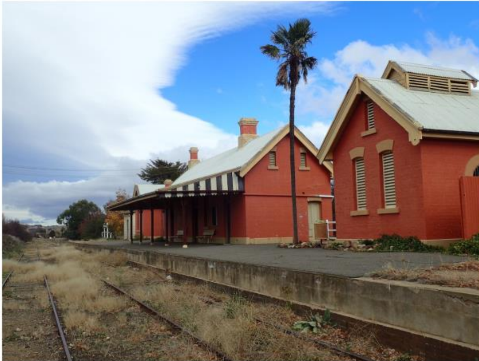
Above: Current condition of Michelago Station.
