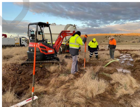
Broken water main, Cooma
