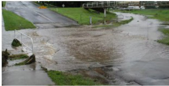
Flooding in Cooma
