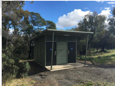
Mt Gladstone Toilet Upgrades
