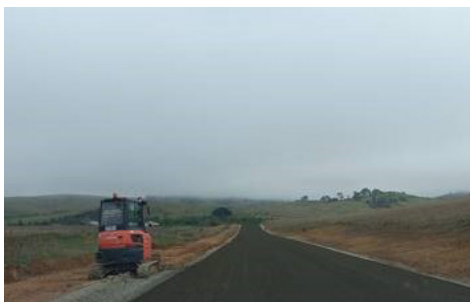
Completed works on Tinderry Road
