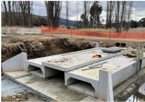
Box culverts to be installed under Michelago Road
