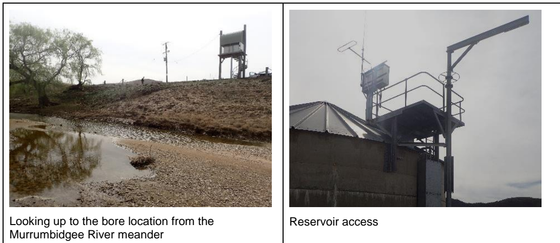
Figure 3-1: Overview of Bredbo Infrastructure.
