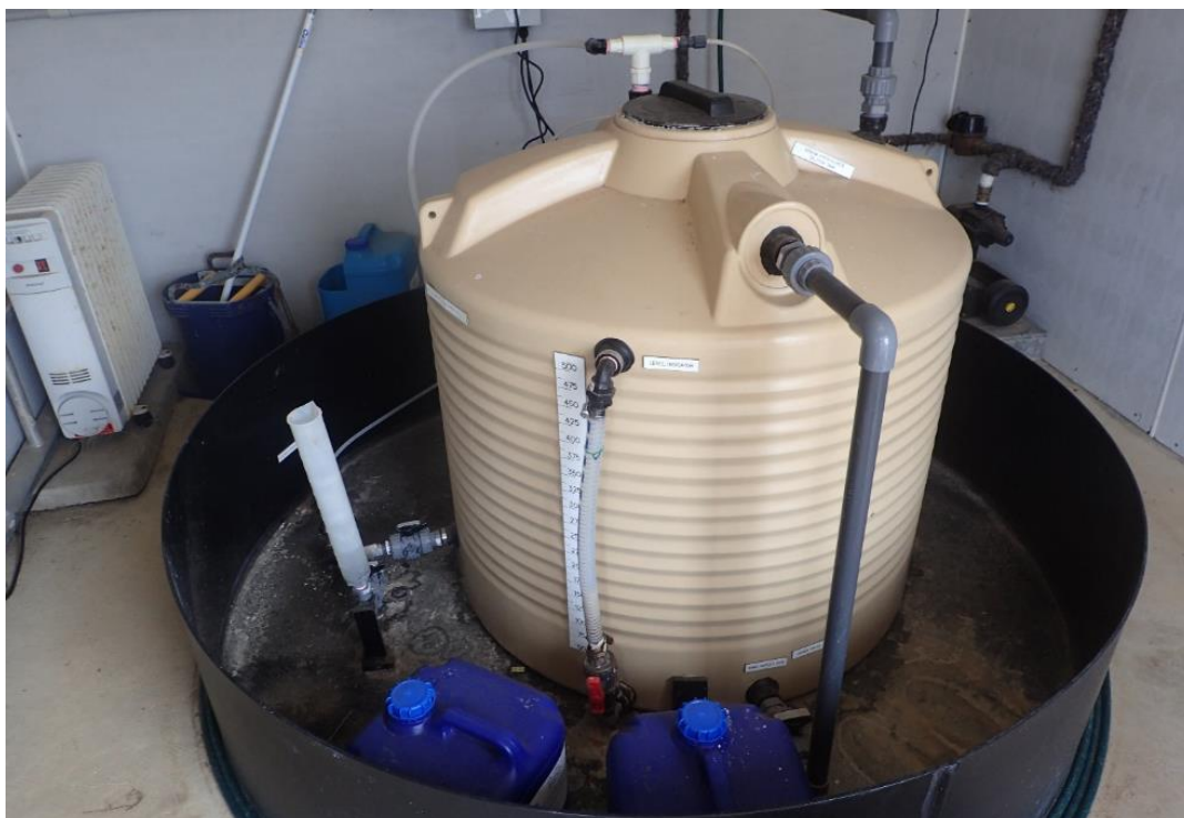
Figure 3-9: Bredbo Hypo Dosing.
