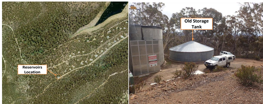
Figure 7-4: Eucumbene Cove Reservoir and Old Storage Tank.
