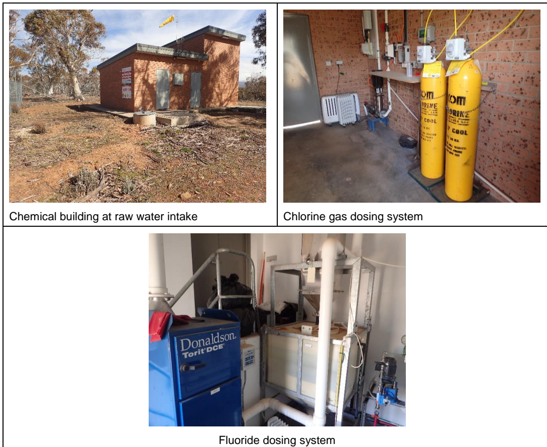
Figure 5-6: Adaminaby Chlorine Dosing System.
