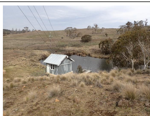
Maclaughlin River water intake and pumping station
