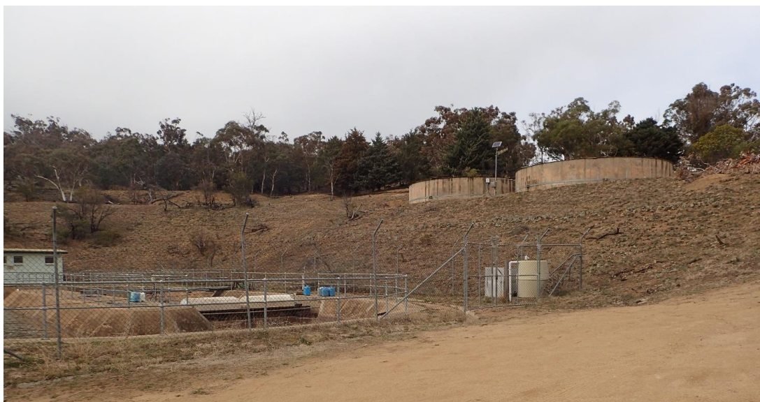
Figure 4-8: Kalkite Reservoirs above the Kalkite STP.
