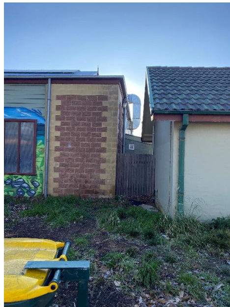
Site Photograph 2 – Western elevation showing location of window to be removed and replaced with new exit door. The building in the foreground is the public toilet block which is on the adjoining lot and will not be impacted by the construction.
