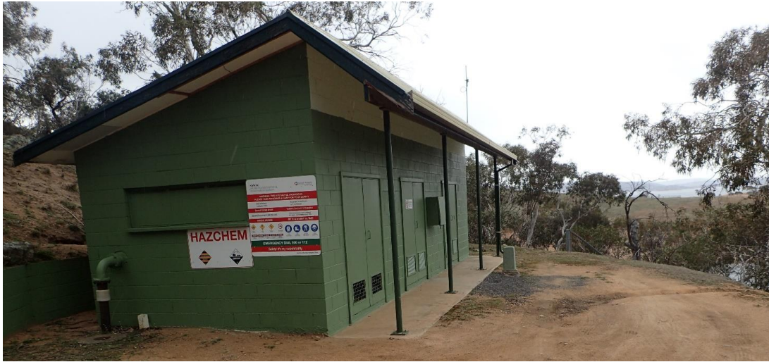
Figure 4-9: Chlorine Dosing System Room.
