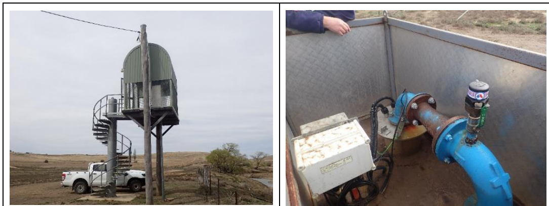
Figure 3-7: Bore Pump Control Structure (Left) and Bore Headworks.
