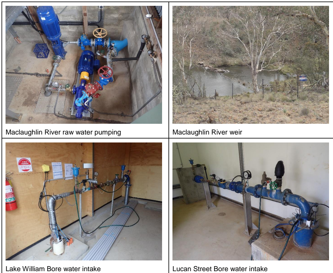
Figure 6-7: Nimmitabel Raw Water Intake and Pumping Infrastructure.
