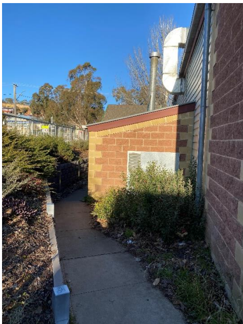
Site Photograph 1 – Eastern elevation of the existing plant room to be demolished. Ducting shown above the plant room will be enclosed in the proposed second storey of the plant room. The path in the foreground will be removed during construction then reinstated upon completion.
