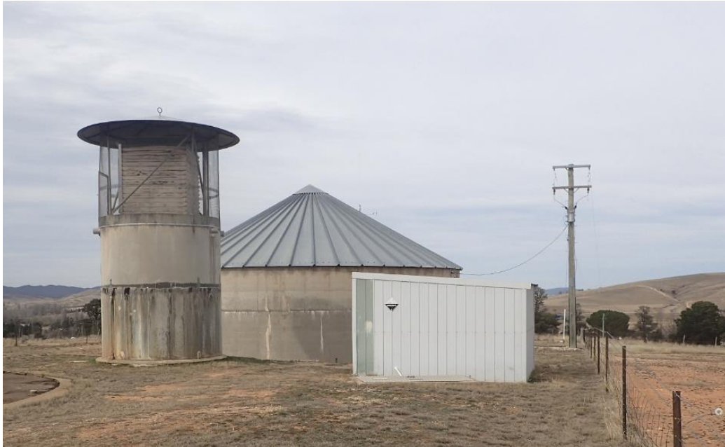
Figure 3-8: Bredbo Reservoir and Aeration Tower.
