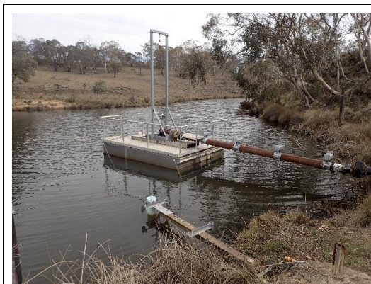
Maclaughlin River Water intake
