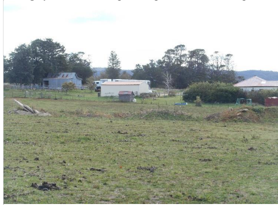
Photograph 4 Lot 1- Existing Dwelling and Sheds – Looking North
