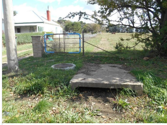
Photograph 2 Existing Culvert Southeast Corner Lot 1
