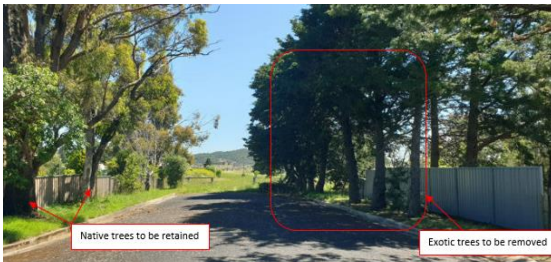
Figure 22: Trees which have the potential to be removed for the construction of the proposed footpath.
