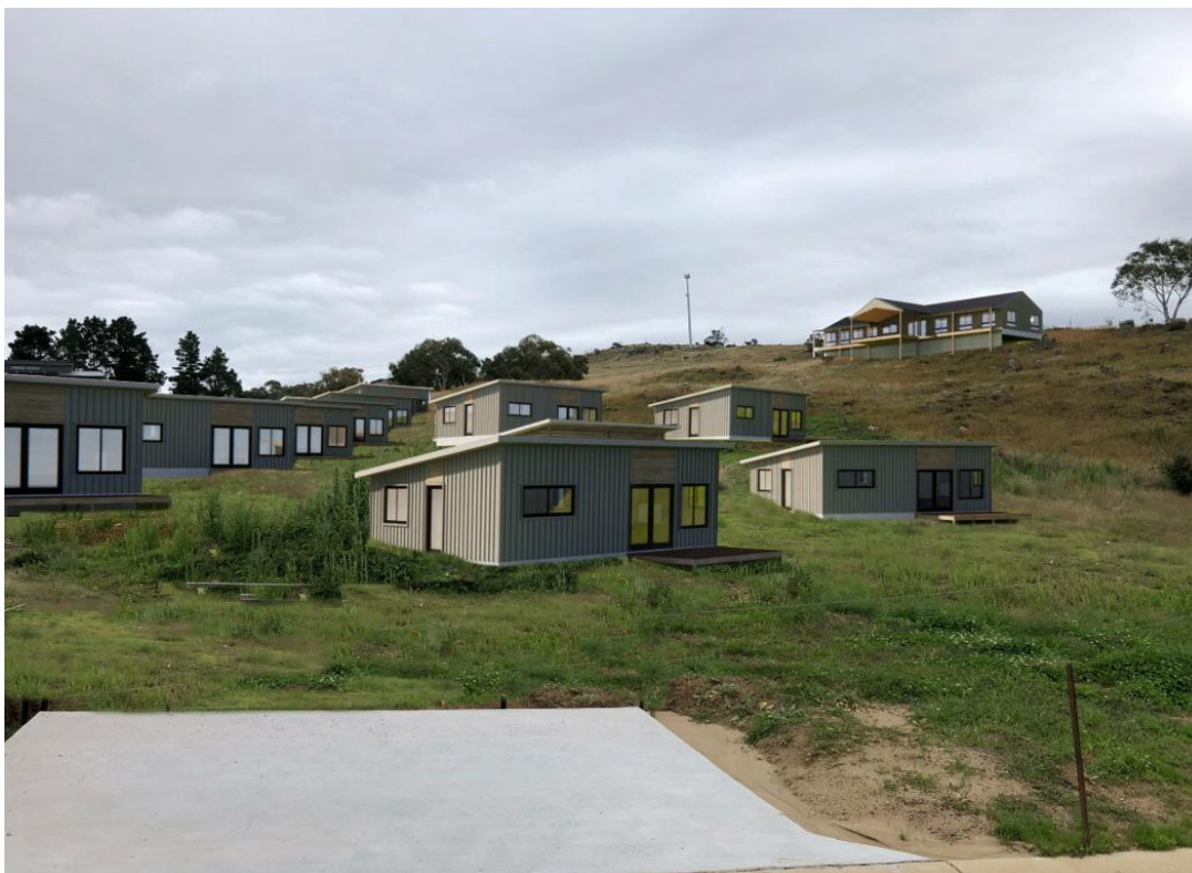
Figure 23: View of the development from Willow Bay Place looking south.
