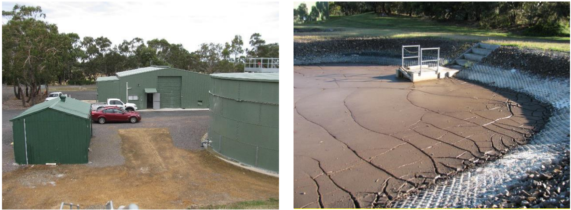
Figure 5 0.6 ML/d Balmoral DAFF main building (left) & Lined sludge drying bed for 23 MLD Hamilton WTP (right)
