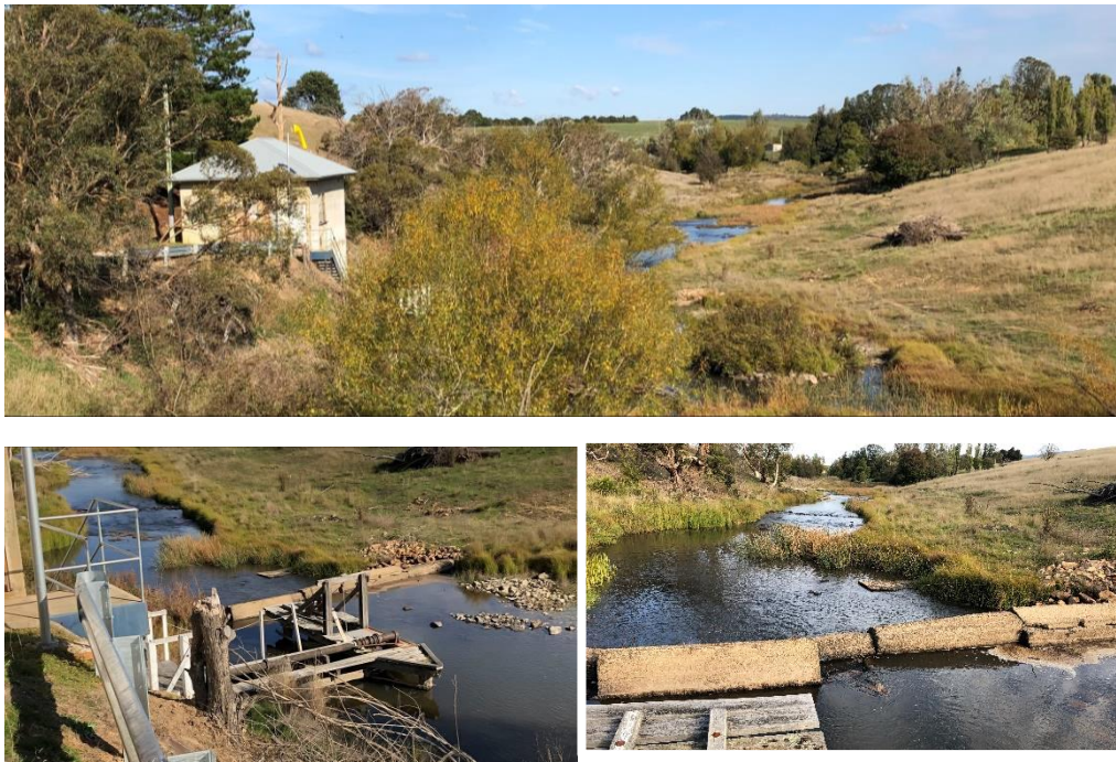
Figure 3 Photo of Delegate water supply Pump station and weir on Delegate River from GHD site visit (16 April 2019)
