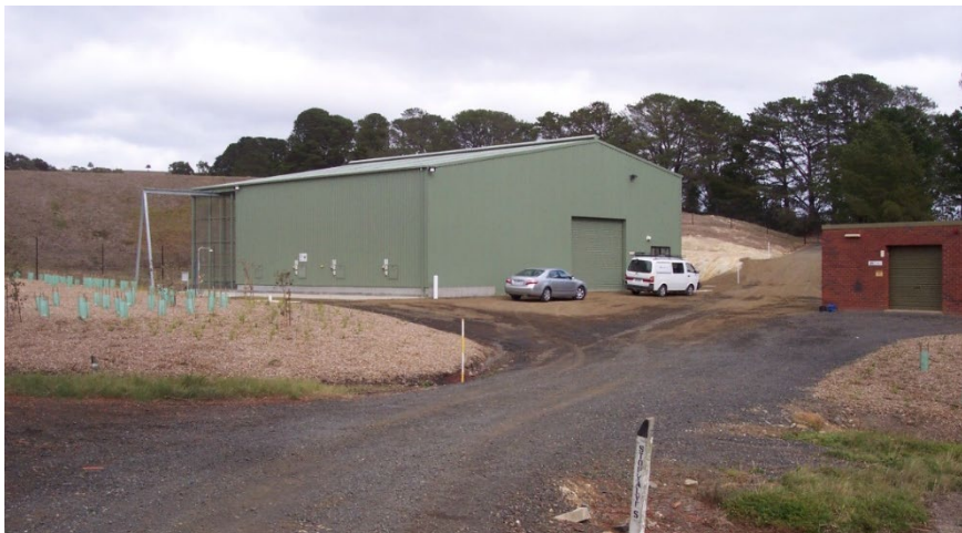
Figure 10 2.5 ML/d Lancefield DAFF water treatment plant main building
