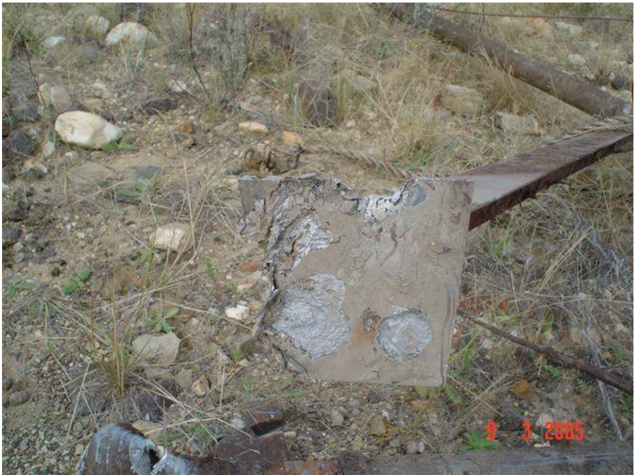
Photo 1. Corrosion of 304 grade stainless steel
