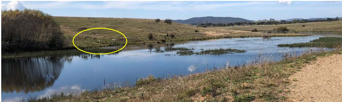
Figure 5 Photo of Coolumbooka Dam from GHD site visit (16 April 2019) showing sheep grazing at edge of dam (circled)
