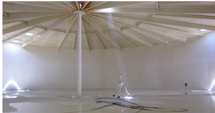
Figure 4. Interior conditions in the Ryan Ranch after cleanout and installation of the PAX mixer.
