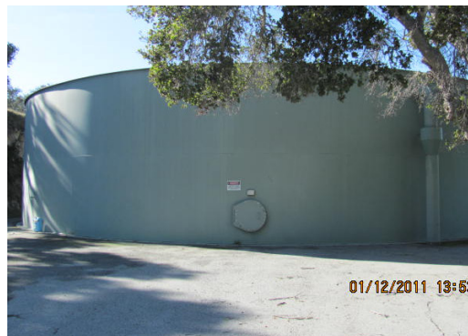
Figure 2. The Ryan Ranch tank is a 500,000 gallon steel ground storage tank
