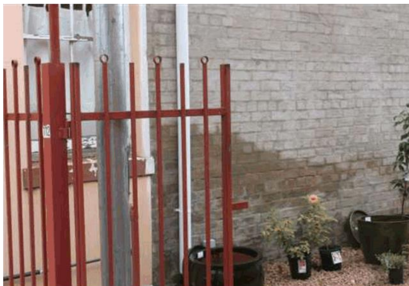
Damp problem on side wall. Note also the surviving period window
