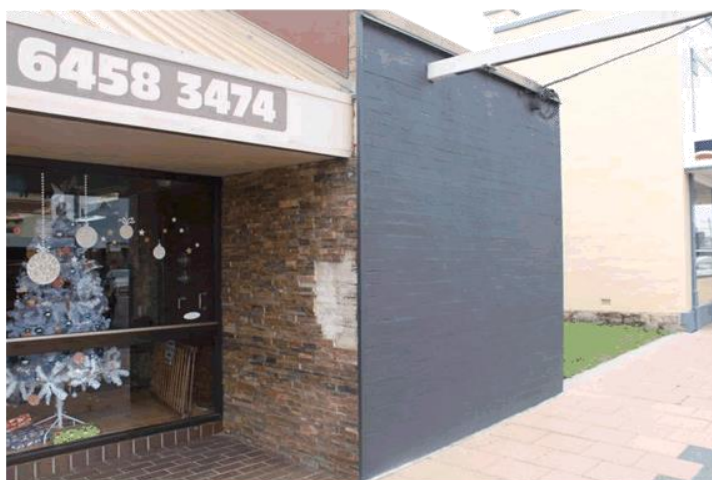
Note missing tiles on wall
