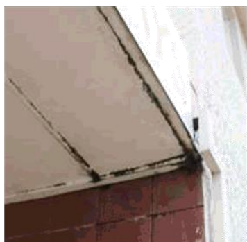
Leaking awning needs repair
