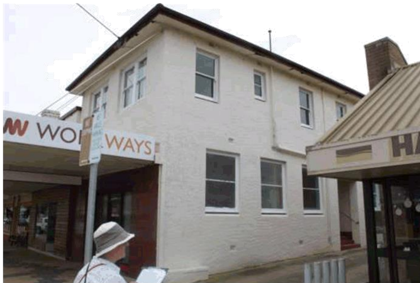
Side elevation showing "Tyrolean" style wall render
