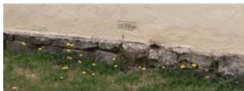
Note the traditional wall vent and stone footings.
