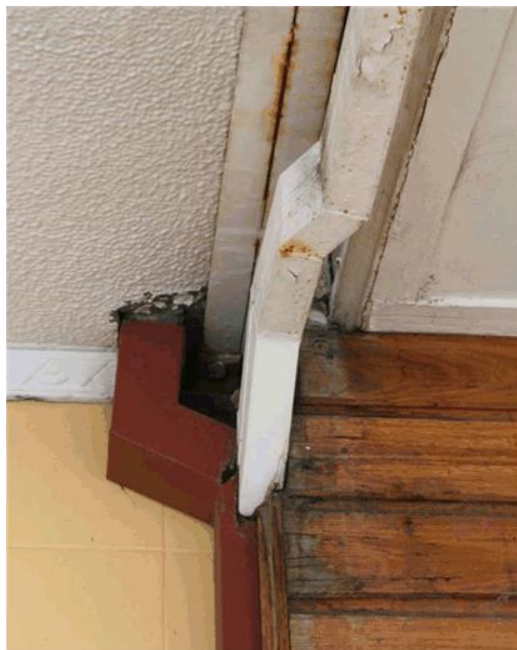
Repair leaking awning and downpipe
