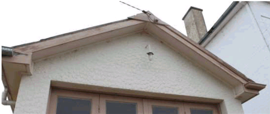
Note damaged barge cap at the fascia.
