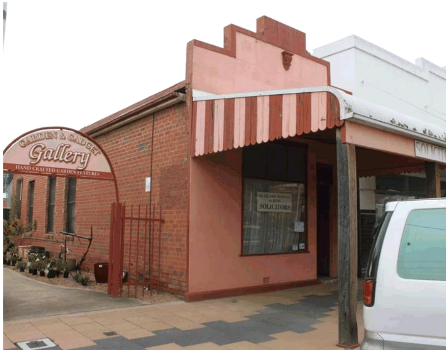
Note damp at lower portion of wall
