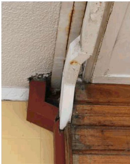
Repair leaking awning and downpipe
