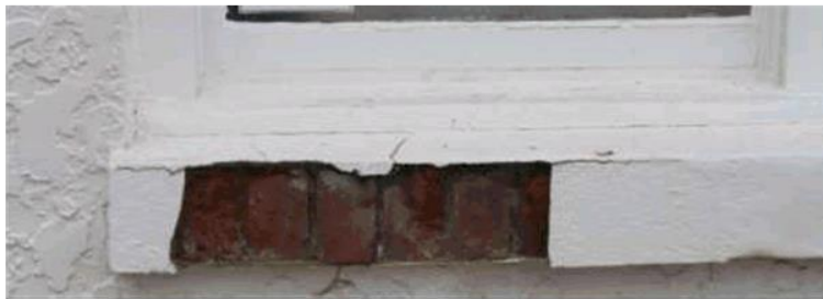
Lost rendering to be repaired – 2016
