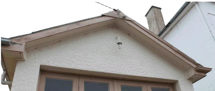
Note damaged barge cap at the fascia.
