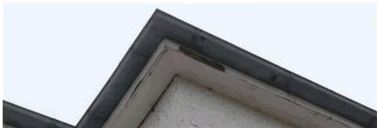
Fascia and soffits to be repaired and painted - 2016
