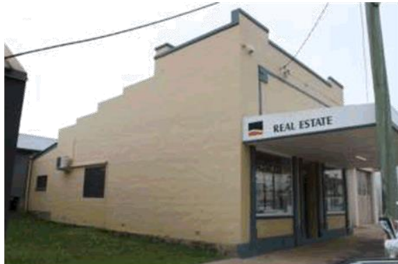
Note the decorative rendering on the face and top edge of parapet.
