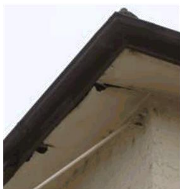
Deteriorating eaves also in need of repair
