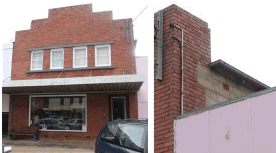
Note cement bricks on side wall
