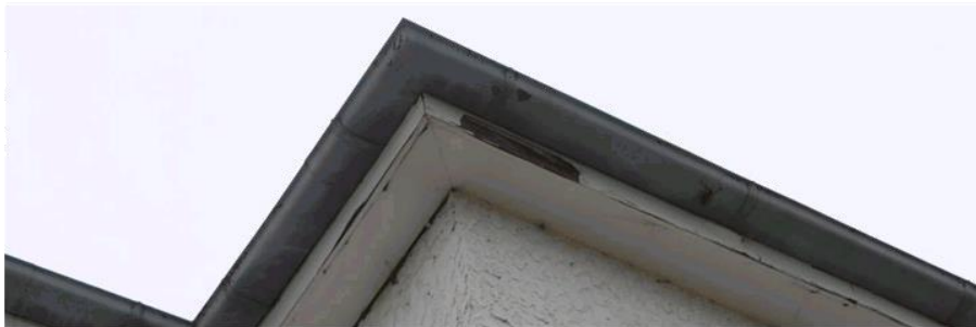
Paint fascias and repair soffits
