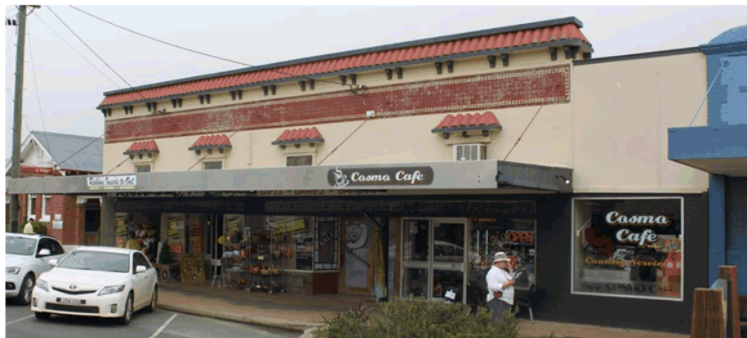
Note efflorescence on tiles on upper parapet
