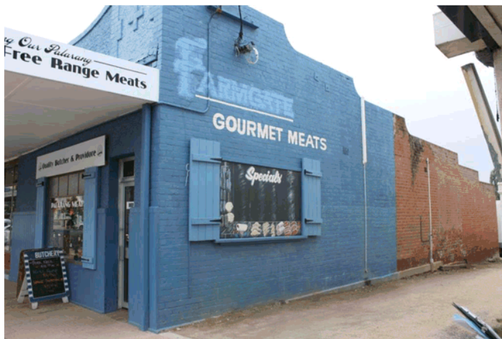
Note damp brickwork at rear of side wall
