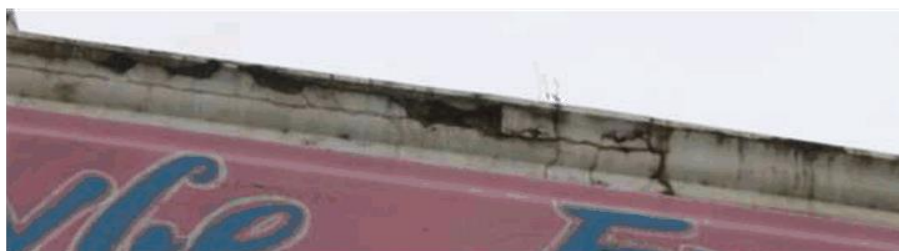
Repair rendering before painting
