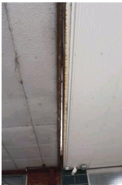
Rusting at edge of awning to be repaired
