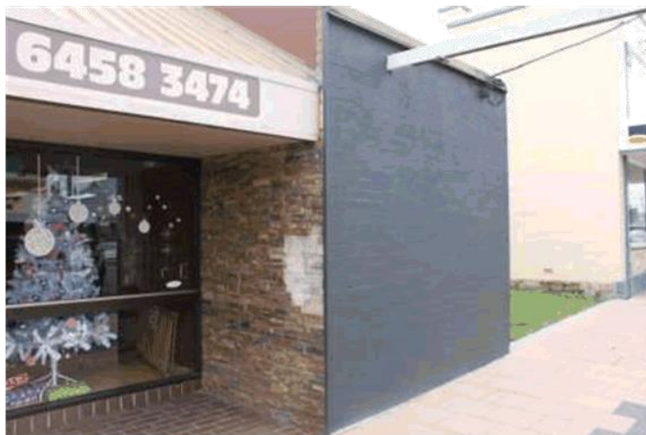
Note missing tiles on wall
