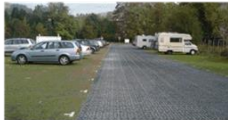
Example of reinforced grass and gravel areas (image source: abg-geosynthetics.com)
