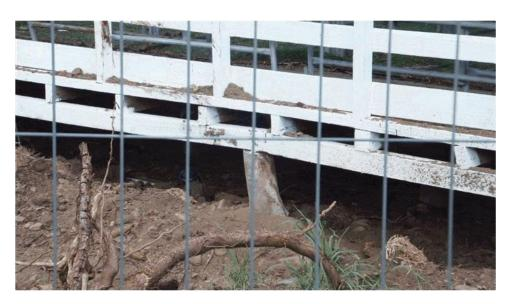
Photograph 8. Example of existing timber stump footings
