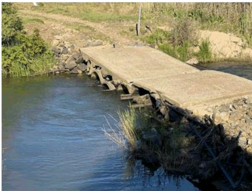
Upstream views of Bairds Crossing – Water velocity estimated at 1.2m/s
