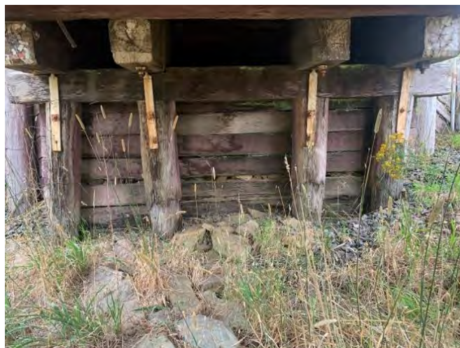
Figure 5-4: View from in between internal girders, all girders were found to be in fair condition with no major deterioration present. Corbels and bent caps were found to be in fair to poor condition throughout with evidence of minor decay present. Brief NDT testing was completed using non-destructive methods, such as EPHOD® Stress Wave Technology. Refer to Appendix A for more information of this type of testing method. Readings for girders were found to be between 300-500 \mu s, Corbels – 400-100 \mu s and caps 300-800 \mu s. This is the time taken for the compression wave to travel across the section of the member tested. This was recorded on most elements and aids in verifying the condition of the elements. The pile tops are in better condition due to the use of horizontal connectors with side plates.
