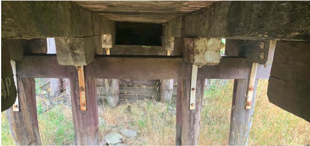
Figure 5-4: View from in between internal girders, all girders were found to be in fair condition with no major deterioration present. Corbels and bent caps were found to be in fair to poor condition throughout with evidence of minor decay present. Brief NDT testing was completed using non-destructive methods, such as EPHOD® Stress Wave Technology. Refer to Appendix A for more information of this type of testing method. Readings for girders were found to be between 300-500 \mu s, Corbels – 400-100 \mu s and caps 300-800 \mu s. This is the time taken for the compression wave to travel across the section of the member tested. This was recorded on most elements and aids in verifying the condition of the elements. The pile tops are in better condition due to the use of horizontal connectors with side plates.
