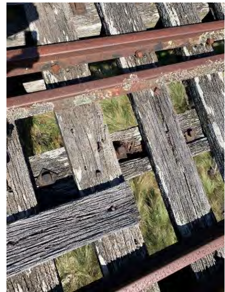
Figure 10-5: View of the walk out standing platform. Platform appears to be in poor to very poor condition with missing/failed members. This would not be safe to stand on. All timber appears to exhibit significant decay.
