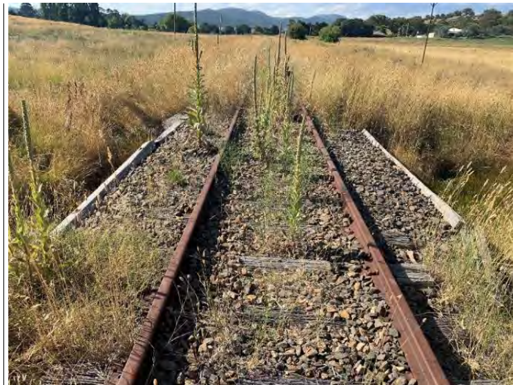
Figure 7-7: The photo above shows the general view down the rail line. Significant overgrown vegetation present through rock ballast and surrounding the substructure. Note: Ballast is 450mm thick.
