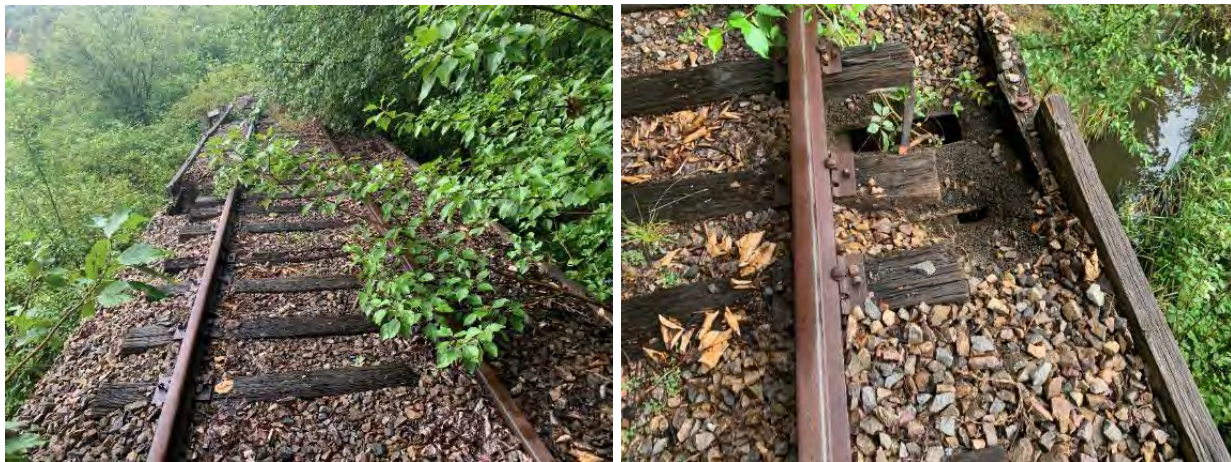
Figure 4-5: The timber transoms were found to be in a very poor (unsafe) condition. The timber ballast tray side walls and rock ballast were in poor condition with erosion of material found in several locations. If the bridge was to be repurposed for pedestrian and cycle use the timber transoms, railway line and rock ballast would need to be removed. Depending on the condition the existing ballast tray side boards they can left in place to act as a kerb/kick rail in the re-purposed bridge. To meet the current standards and Australian codes; vertical balustrade panels and a 1.4m high cycle rail will need to be installed. Note: Significant vegetation growth. The ballast tray will provide a great subgrade for the walking track.
