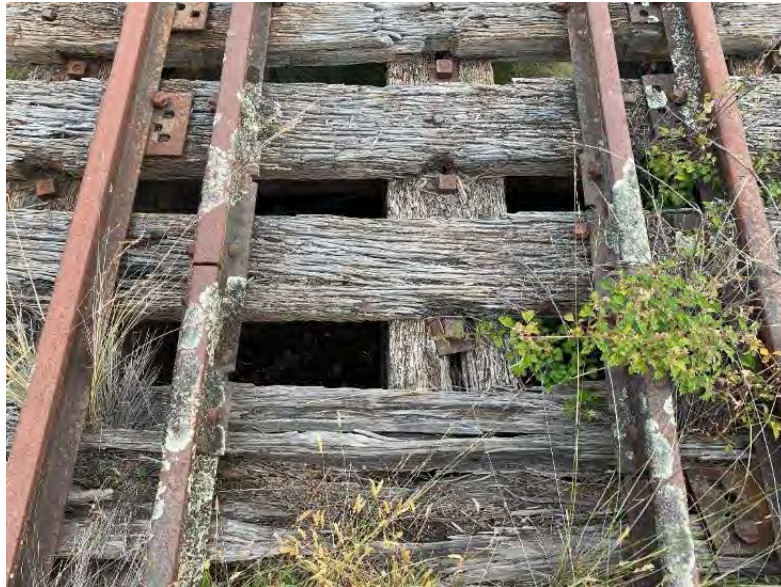
Figure 11-7: View of the bridge open deck, transverse sleepers were found to be in poor to very poor condition with significant decay, cavities and severely damaged members present throughout. It was noted that the vertical connections to the top girders were seen to funnel moisture and increase the moisture content present in both elements causes significant decay. When the moisture content exceeds 22%, timber consuming fungi are activated, and the decay process begins. Top girders were found to be in poor to very poor condition.
