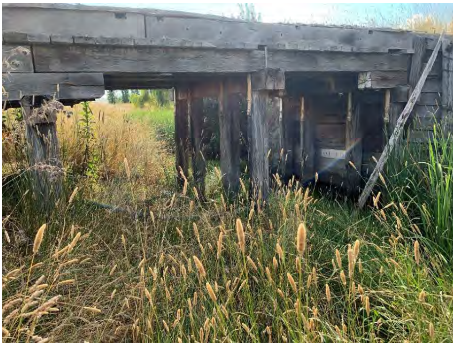
Figure 6-1: General view of Lobbs Hole Creek Bridge from the side of the bridge. The Creek that flows underneath span 1 at the time of inspection was flowing very slowly/still. The configuration of the bridge is a girder under and consists of 3 spans, 2 abutments and 2 pile bents. The span length is 3m equating to a total length of 12m. Note: abutment 1 and abutment corbels as does one of the bents.
