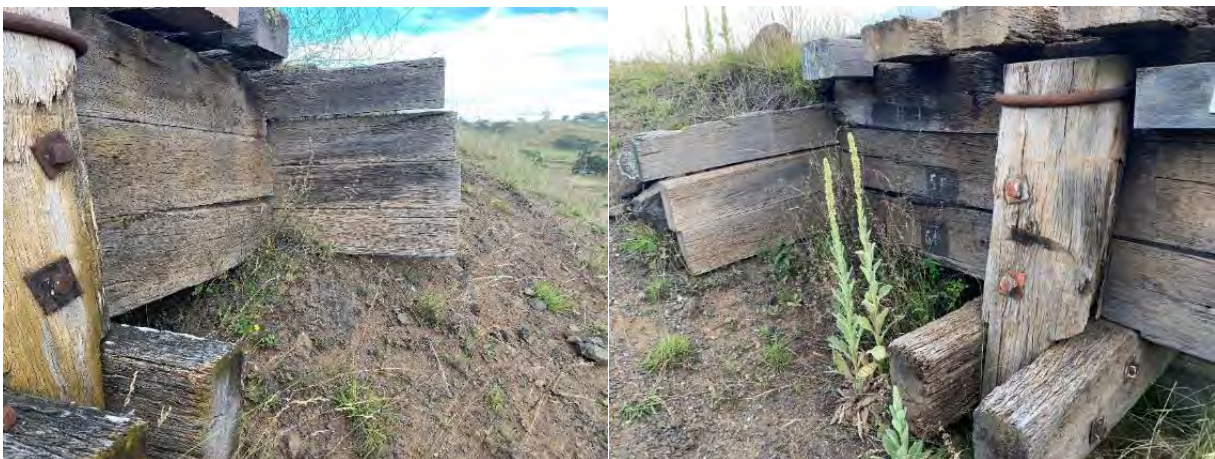
Figure 11-4: The images above show the condition of the breast wall at AB2. The abutment sheeting was found to be in fair condition with minor decay of the sapwood present. The headstock ends were in poor condition with decay and cracking present.
