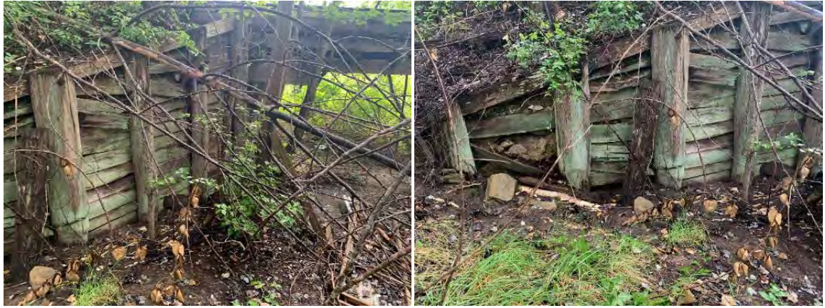
Figure 4-8: The timber wingwalls have undergone significant deterioration with timber sheeting completely rotted and failing in several locations. Due to this the walls' ability retain the approach fill material is poor leading to erosion and excessive loading.
