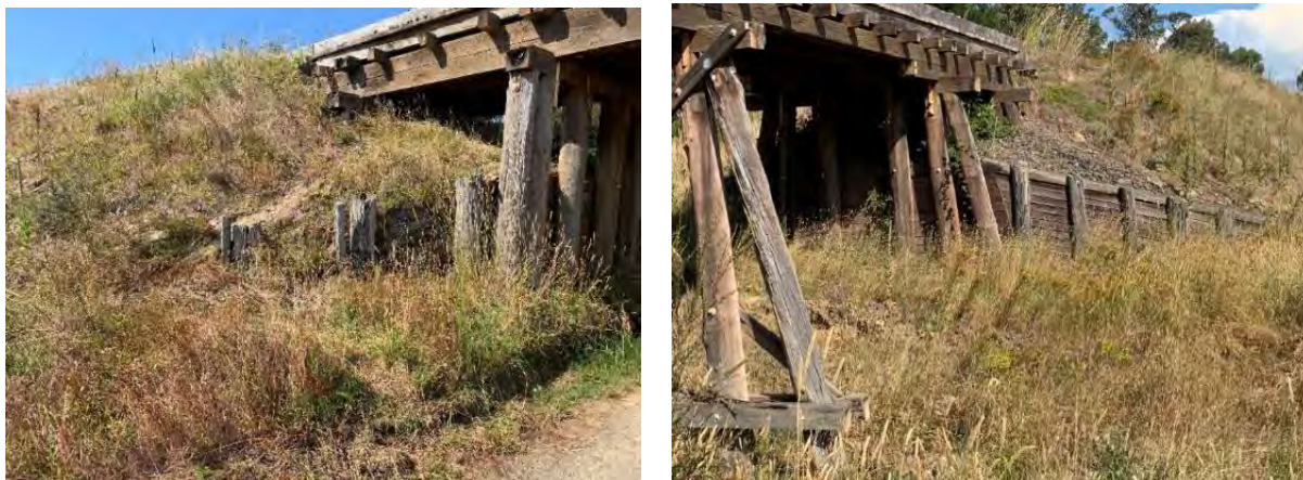
Figure 8-4: The images above show the condition of the breast wall at PB1 & 4. The left photo shows the breast wall at PB1 to be poor to very poor condition with significant decay in timber elements present, surrounding overgrown vegetation and erosion of back fill material. The right image shows the breast wall at PB4 to be in fair to poor condition, it was noted that the back fill material had forced the wall to “lean” forward. Note: Severely decayed batter pile at PB3.
