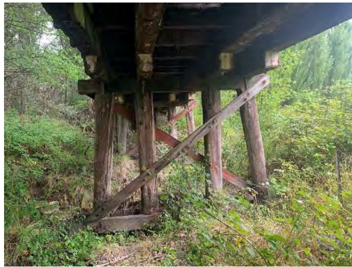
Figure 4-2: View of the typical timber pile bent configuration. The bent is comprised of 4 driven piles, single timber head stocks and corbels. The bent is also supported by a double cross bracing system with sashes at halfway and timber wales at the bottom. Overall, the timber bents were found to be in a poor to very poor condition. Note the surface brown rot fruiting bodies on the faces of some of the cross braces -orange brown colour.
