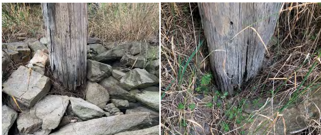
Figure 5-2: General configuration of each pile bent. Large vegetation growth and cobbles located around the base of piles. All piles were found to be in very poor condition with large splits and sapwood decay are present in majority of piles, predominately at ground level. Excess vegetation growth leads to an increase in moisture content within timber members resulting in accelerated decay.
