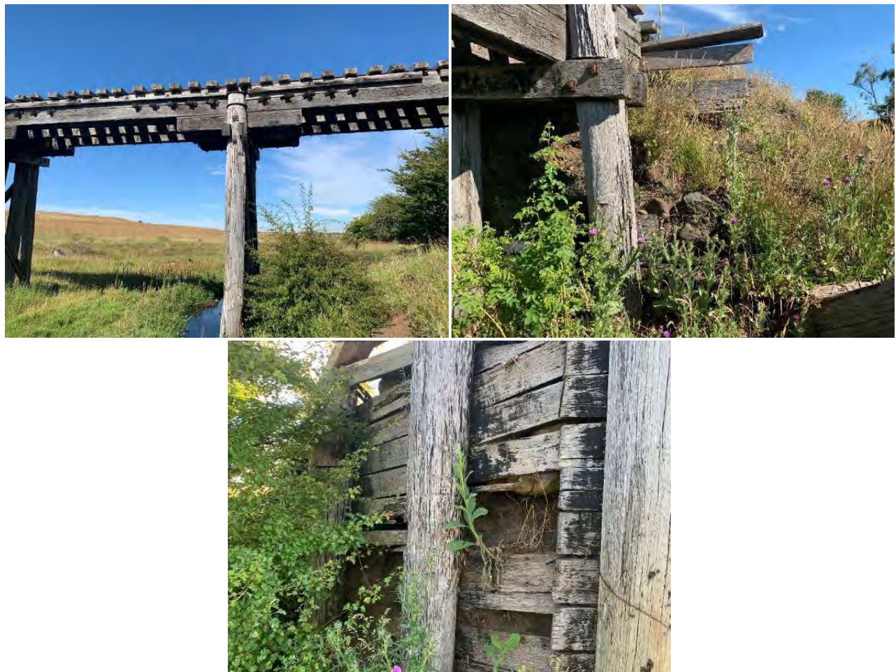
Figure 9-5: Large amounts of sapwood decay is present throughout the structure piles. It is recommended that this is monitored and removed appropriately.
