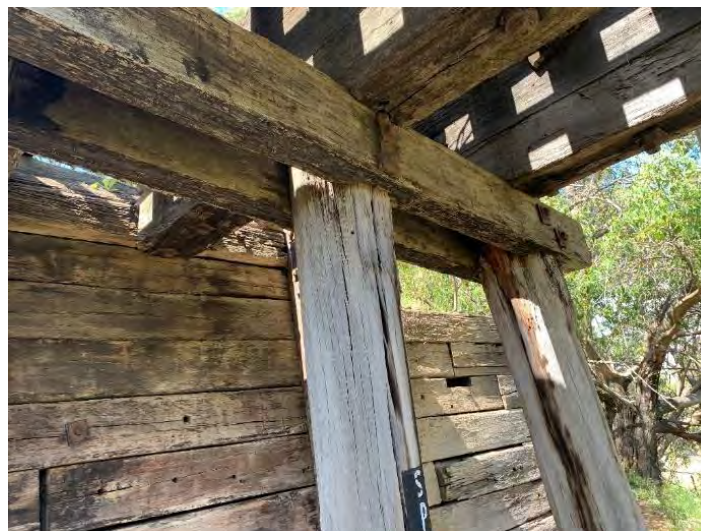
Figure 10-4: The images above show the condition of the split headstocks and the abutment breast wall. The headstocks were found to be in poor to very poor condition, exhibiting significant decay. The breast wall is in poor condition with missing members and weathered elements with splits and cracking throughout. Note: major vertical crack down middle pile exposing bright wood and accelerating decay. Typically, these decay cracks are initiated by fastener systems
