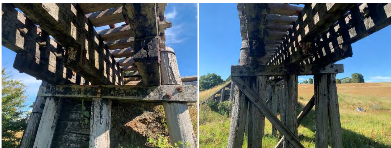
Figure 9-3: The images above show the substructure configuration. It is seen that double stacked girders have been used in addition to split headstocks and corbels. Both images show significant water stains and decaying of corbel ends. The left image identifies a large cavity present in the end of corbel 1 AB1. It was noted that AB1 sheeting has failed.
