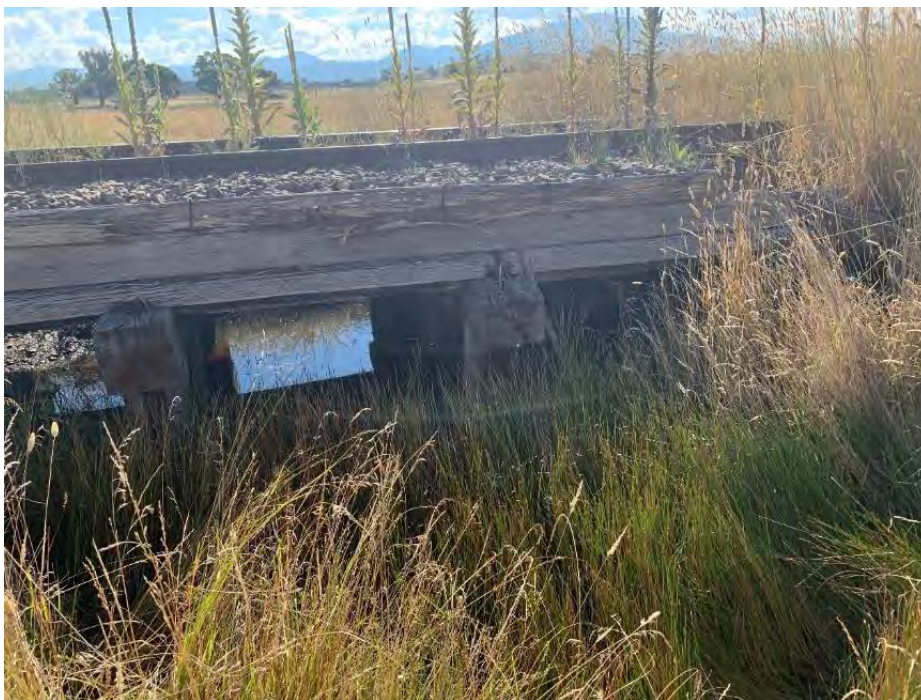
Figure 7-1: The image above shows a general view of the 7m minor bridge (Williamsdale Rd). The consists of 3 spans each span is 2m in length, substructure includes 2 pile bents and 2 abutments that each have 4 driven piles, a pile cap and 4 girders. At the time of inspection there was water approximately 0.5m deep in Spans 1-3. There is a large amount of vegetation growth around the substructure which keeps the moisture content high in the timber. When the moisture level in the timber is above 22%, decay-causing fungi can start to grow; when the moisture content drops below this level, the fungi become dormant, and decay will be arrested until the moisture content rises again.
