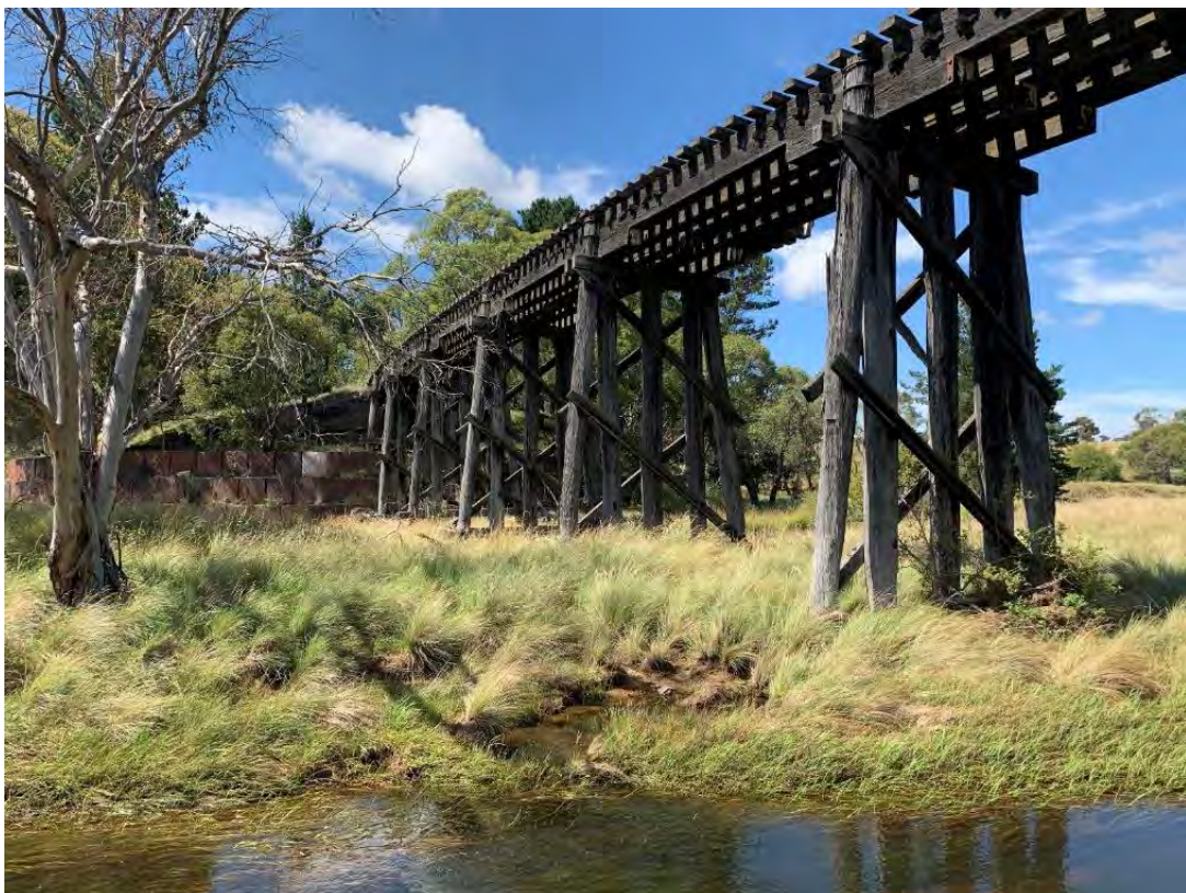
Figure 10-1: General view of MacLaughlin River Bridge from abutment 2 looking towards abutment 1. The timber bridge is 8 spans long and approximately 60 metres in length (7.5-8m spans). Note MacLaughlin River runs underneath span 3 and is approximately 3m wide and 0.7m deep. It was also noted that the bridge curved left and had appropriate camber. Note the double cross bracing on the bents as well the absence of a sash brace.
