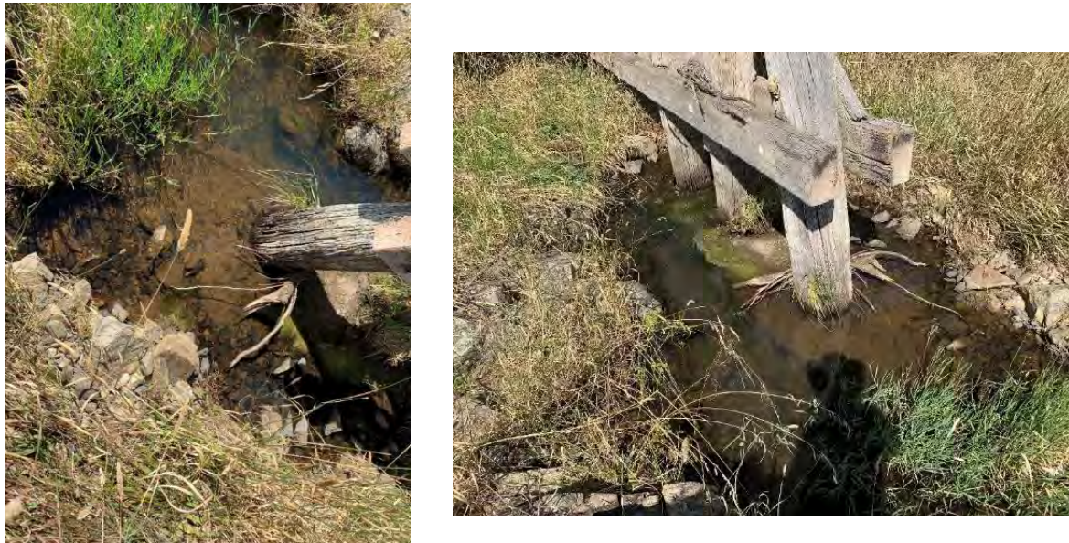
Figure 8-3: General view of pile bent 3 bearing on a concrete sill, piles were found to be in poor to very poor condition. The bottom sections of the timber piles were determined to be a ‘hotspot’ for decay and determined to be an ideal area to test using non-destructive methods, such as EPHOD® Stress Wave Technology. The timber piles were estimated to produce SWT data ranging between 300-1400 \mu s. Readings above 700 \mu s indicates that there is significant decay present and are required to be monitored. Reading of above 1000 \mu s indicate severe decay is present resulting in the member being unable to support its own dead load.
