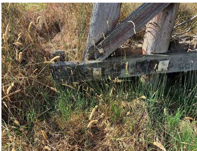
Figure 8-6: A view of a cross bracing plank connection. Plank was found to be in very poor condition as the end has completely decayed away to the connection point. Timber wales were found to be in poor condition with significant water stains and decay present throughout.
