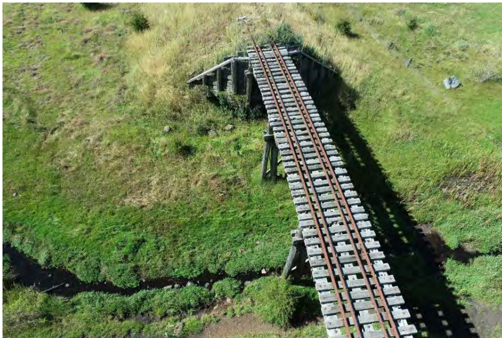
Figure 9-1: General view of Bobundara Creek Bridge from abutment 1 looking towards abutment 2. The timber bridge is 3 spans long and approximately 22.5 metres in length (7.5m spans). Note Bobundara creek runs underneath span 2 and is approximately 1m wide and 1ft deep. note the inner guard rail to prevent derailment leading to the train going off the bridge when train operations were occurring.
