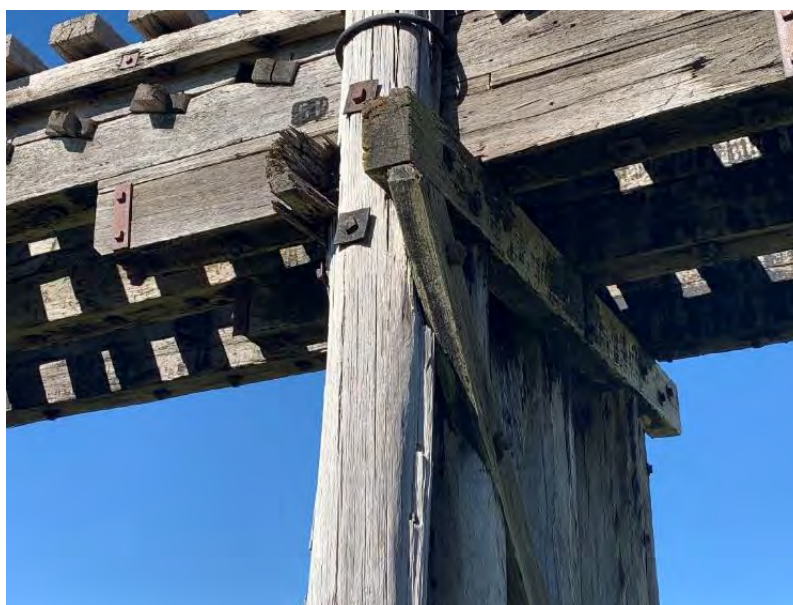
Figure 9-4: The images above show the condition of the split headstocks. The majority of headstocks were found to be in poor to very poor condition. The left member in the image above is completely decayed through the end and in very poor condition.
