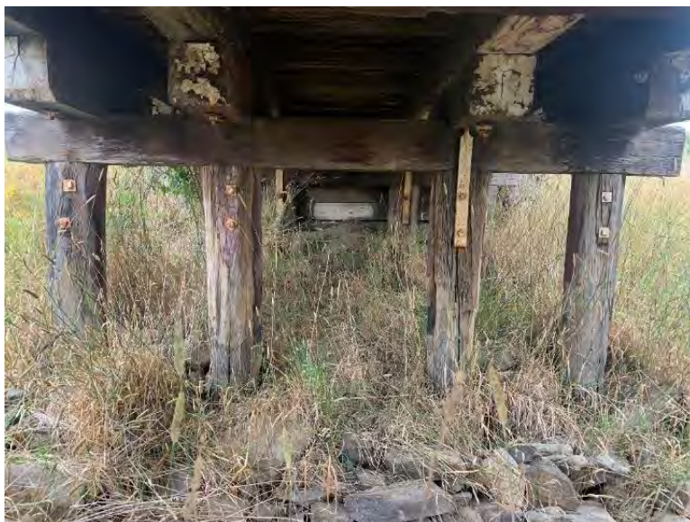
Figure 5-2: General configuration of each pile bent. Large vegetation growth and cobbles located around the base of piles. All piles were found to be in very poor condition with large splits and sapwood decay are present in majority of piles, predominately at ground level. Excess vegetation growth leads to an increase in moisture content within timber members resulting in accelerated decay.
