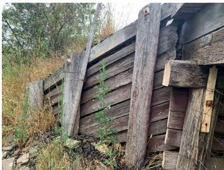
Figure 5-6: A view of abutment wingwall. The wingwall was found to be in fair to poor condition with minor deterioration present throughout all components. Minor deformation was present at top of wall due to bearing load of ballast.
