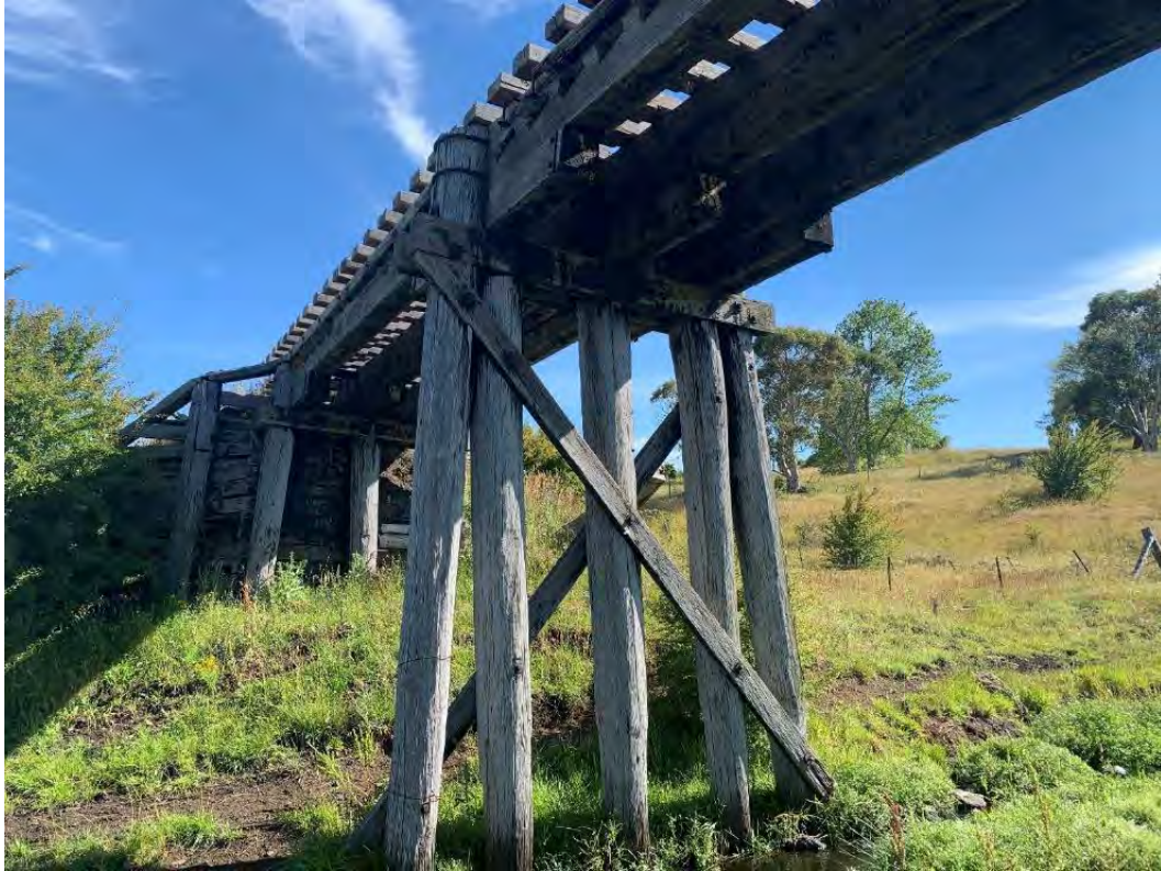
Figure 9-2: View of the timber pile bents configuration. PB 2 and 3 comprise of 5 driven piles (3 Plum piles directly under the girders and 2 batter piles on either side). Pile bent 2 and 3 are supported by cross bracing. The two abutments do not contain the cross bracing and are support by timber sheeting to retain backfill. It was noted that the bottom section of several posts has started to undergo decay. This can be expected due to the timber posts being exposed to increased moisture in overgrown vegetation, debris, and the nearby creek. Once the moisture content in the timber elements reaches 22%, decay causing fungi are activated and the decay process begins. Overall, the timber bents were found to range from poor to very poor condition.
