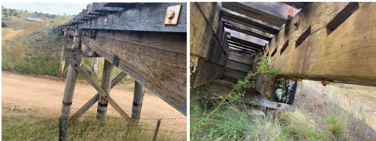
Figure 11-6: A view of girders formation and condition. Girders were found to be in fair to poor condition, the left photo shows a horizontal crack that is seen to be progressively increasing in size. The right photo shows sapwood decay of the internal girders.
