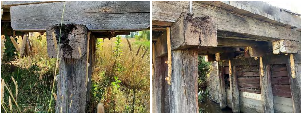
Figure 6-6: Above photos show the ends of the pile bent caps at PB1&2. Minor deterioration and cavities were found at all ends of caps. Overall, the caps were in poor condition. Brief NDT testing was completed at the mid length using non-destructive methods, such as EPHOD® Stress Wave Technology. Refer to Appendix A for more information of this type of testing method. Readings for bent caps were found to be between 200-1000µs. This is the time taken for the compression wave to travel across the section of the member tested. This aided in verifying the overall condition of the elements.
