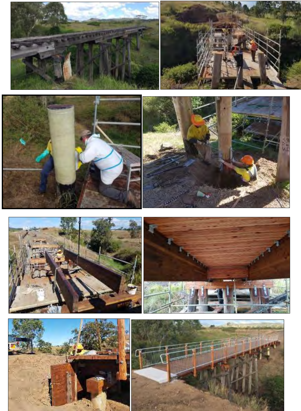
Figure 12-9: The photo series above demonstrates an Option 2 type of fix that was done for Jimmy Gully Bridge along the BVRT. The existing poor condition superstructure was removed, and the piles were repaired or posted with new section. New glulam back wall, caps, girders, and deck system were installed utilising a horizontal connection detail.
