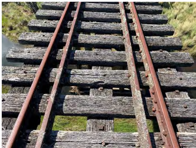
Figure 10-6: Top view of bridge open deck. Transoms and girders can be seen to be in poor to very poor condition, with significant deterioration present in all elements. This is seen to be caused by the vertical connections used in construction. If not sealed appropriately they are seen to funnel water and become moisture traps, when moisture content within timber exceeds 22%, decay causing fungi are activated and the decay process begins. Note: Large cavity around vertical connection in right side photo.
