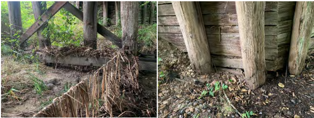
Figure 4-4: The bottom sections of the timber piles were determined to be a ‘hotspot’ for decay, this is caused by the moisture retained by debris increasing the moisture content in timber members. Sapwood decay in the timber piles is photographed on the right-hand side. Refer to Section 4.1 below for a full list of recommended repair options for refurbishment to a pedestrian/cycle bridge.
