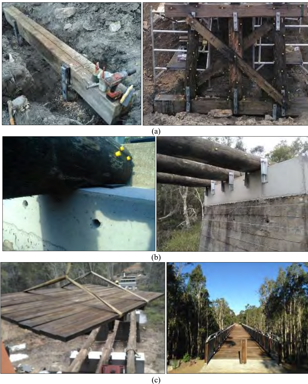
Figure 12-3: The above photo series demonstrates Option 2 type of fix (hardwood) used for the construction of two Mary to Bay Rail Trail Bridges. Seen above in photo (a) is the construction of a frame bent using an intermediate cap which was installed on top of the existing pile stubs. This allowed the hardwood posts, cross bracing, and cap to be installed at the correct reference height. Also note the yellow plugs that indicate that Decaystop® rods have been installed. Photo (b) shows the girders being installed using a horizontal connection system and a rubber liner between the timber girder and concrete pier. In photo (c) the pre-panelised deck is installed along with the modulus handrail and cycle rail system.
