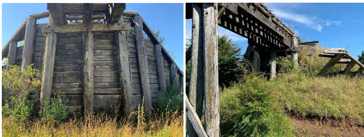
Figure 9-6: A view of two pile defects located at AB1 and PB2. The left image shows decay of sapwood forming a vertical cavity. The right image shows significant deterioration of sapwood (Peeling off).
