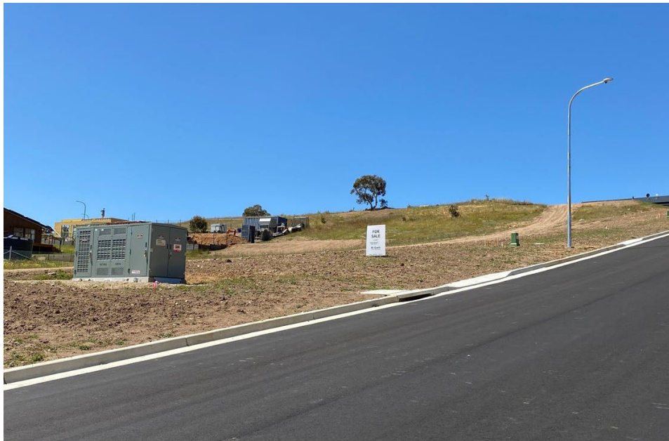
Figure 3: View of Site looking North The Substation is in the South-East Corner of the Site
