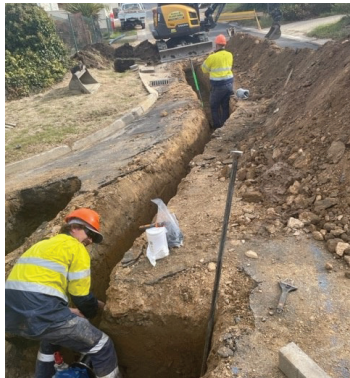
Giwang Street watermain replacement–SMRC water and wastewater are currently renewing the existing 100 mm water main running along the southern side of Giwang Street. Renewal includes three water hydrants, two stop valves, six short services and one long service
