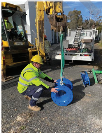
Cooma Water Treatment Plant–A new flow metre was recently installed at the Cooma WTP
