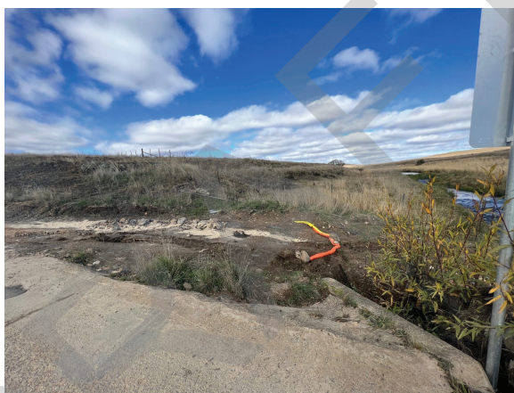
Boom and absorbent material placed to absorb an oil spill
