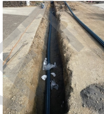
Giwang Street watermain replacement–SMRC water and wastewater are currently renewing the existing 100 mm water main running along the southern side of Giwang Street. Renewal includes three water hydrants, two stop valves, six short services and one long service
