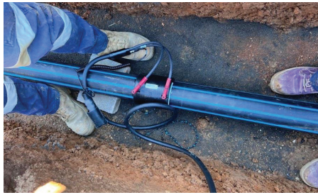
New water main is 100mm HDPE piping using electrofusion welding technology
