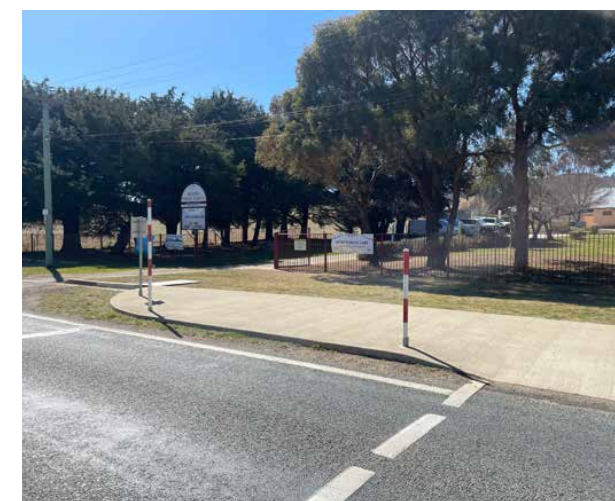
View of existing crossing in front of Bredbo Public School
