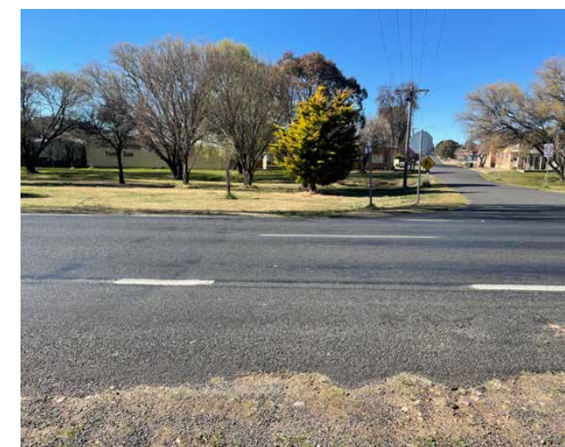
View of Oliver Street crossing point
