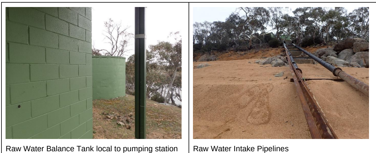
Figure 4-7: Raw Water Intake Pipeline and Balance Tank.
