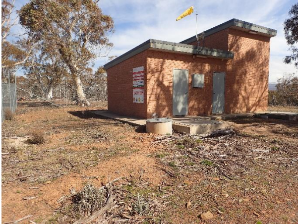
Chemical building at raw water intake
