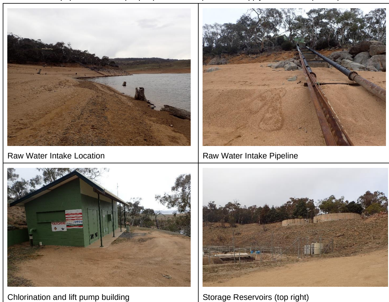
Figure 4-1: Overview of Kalkite Infrastructure.
