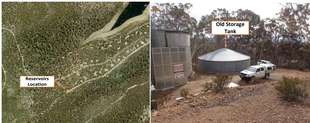
Figure 7-4: Eucumbene Cove Reservoir and Old Storage Tank.
