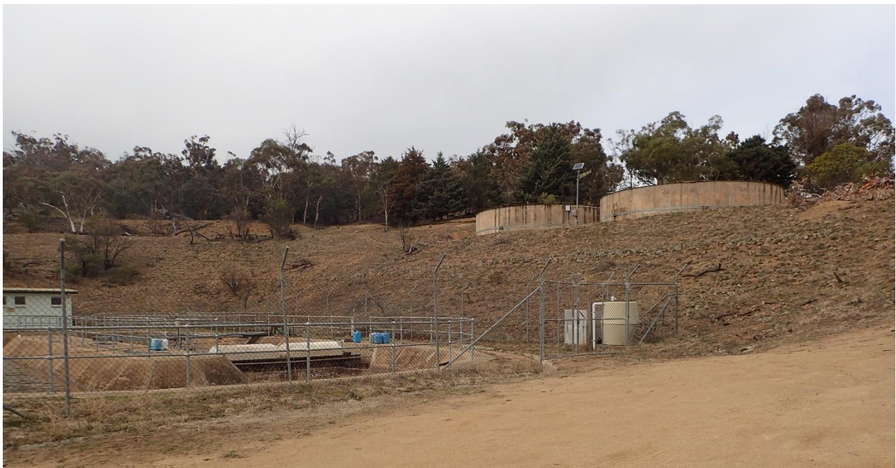
Figure 4-8: Kalkite Reservoirs above the Kalkite STP.
