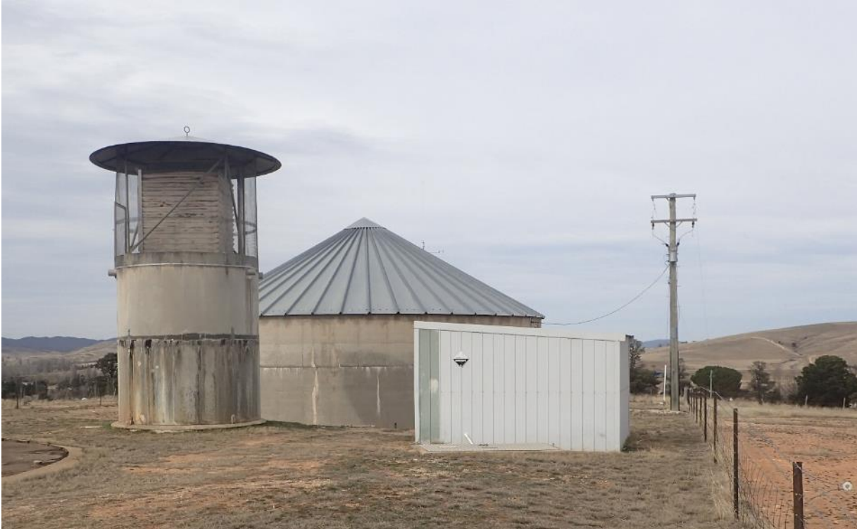
Figure 3-8: Bredbo Reservoir and Aeration Tower.
