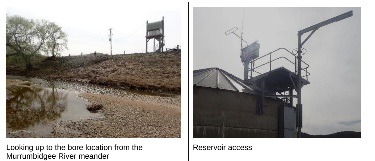
Figure 3-1: Overview of Bredbo Infrastructure.
