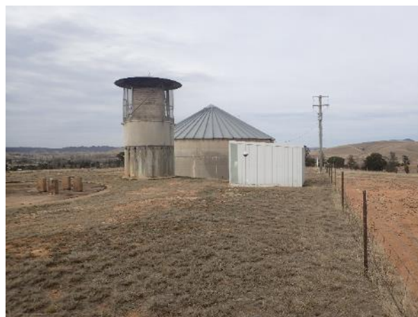
Aeration tower and reservoir
