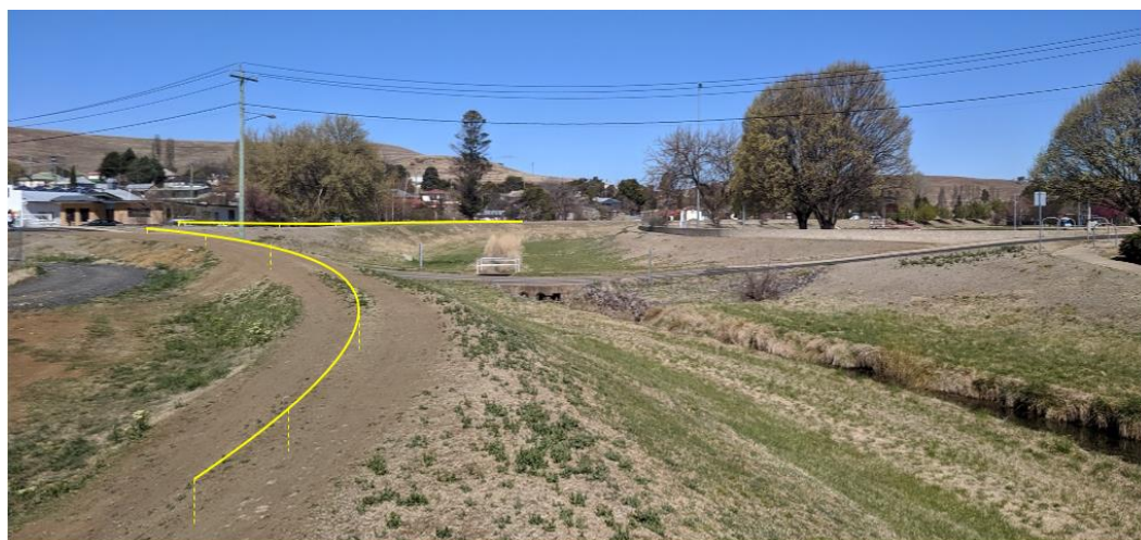
Visualisation of levee raised by approximately 0.3 m (yellow lines) near Commissioner Street. The average raised amount is 0.2 m but some sections will be around 0.3 m higher.
