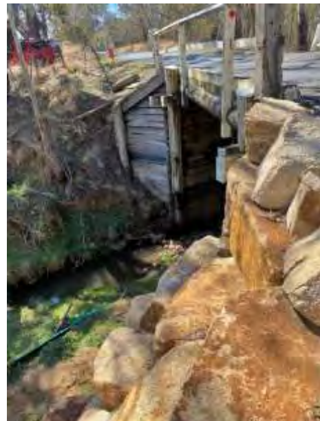
Plate 4: Looking across the bridge with erosion present along steep creek bank (South)
