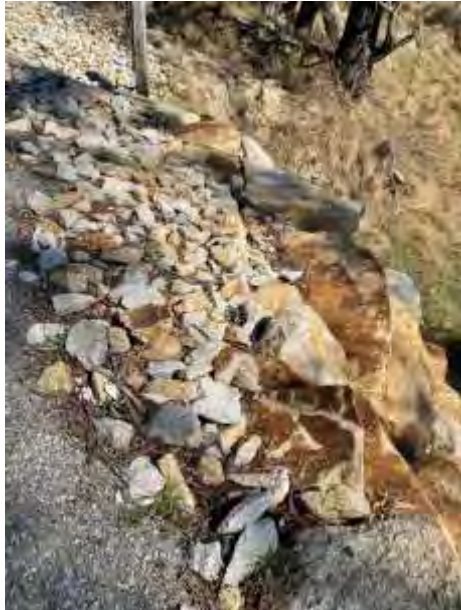
Plate 5: Rock retaining wall along north side of the bridge/creek bank (Northeast)
