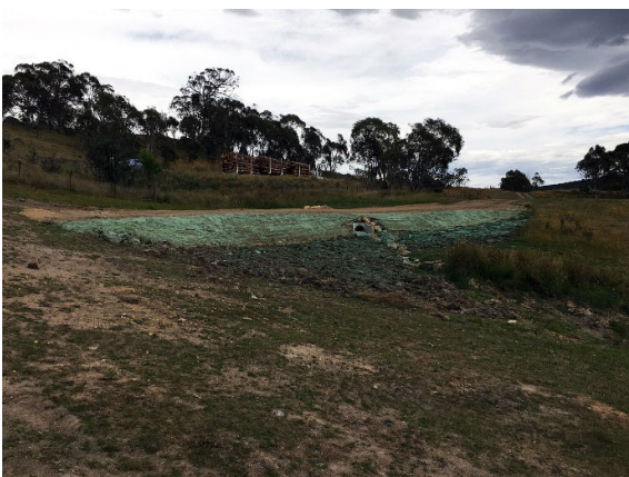
Drainage line track crossing and culvert at the Lake Wallace offset site. Edge drains and jute logs upstream of the culvert, and jute mesh and energy dissipation rocks below the culvert have been installed.
