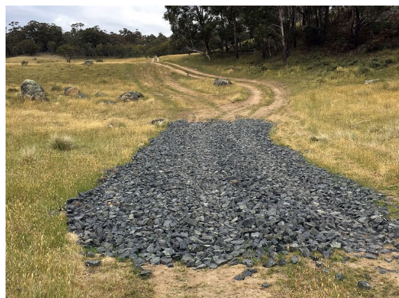
Rock on access track to flow monitoring station to protect environmental and cultural values at the Lake Wallace offset site.
