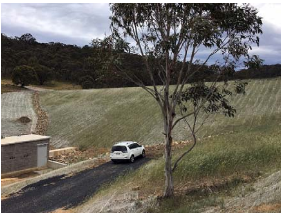
Lake Wallace dam wall and surrounds stabilised and seeded at the end of winter 2016
