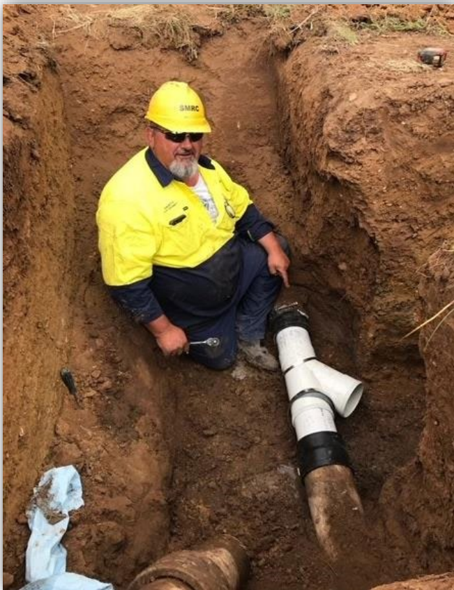
Photo 5 Council water and wastewater team repairing mains
