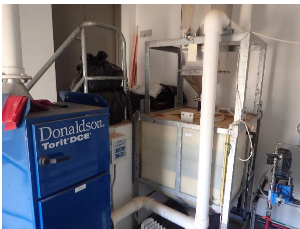
Sodium fluoride dosing system
