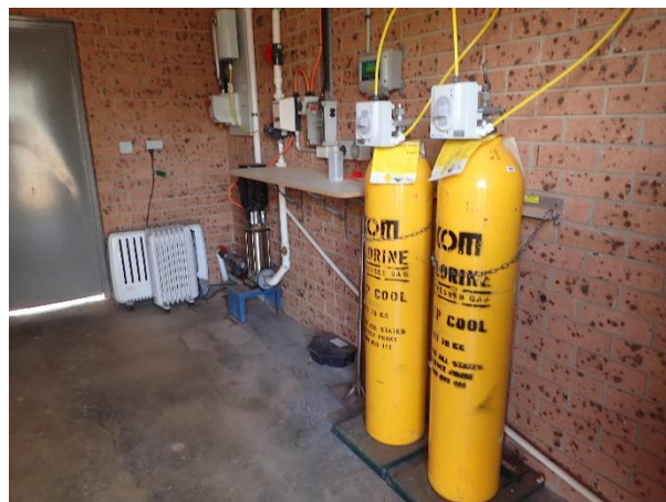
Chlorine gas dosing system
