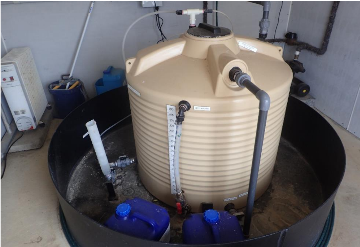
Figure 3-9: Bredbo Hypo Dosing.
