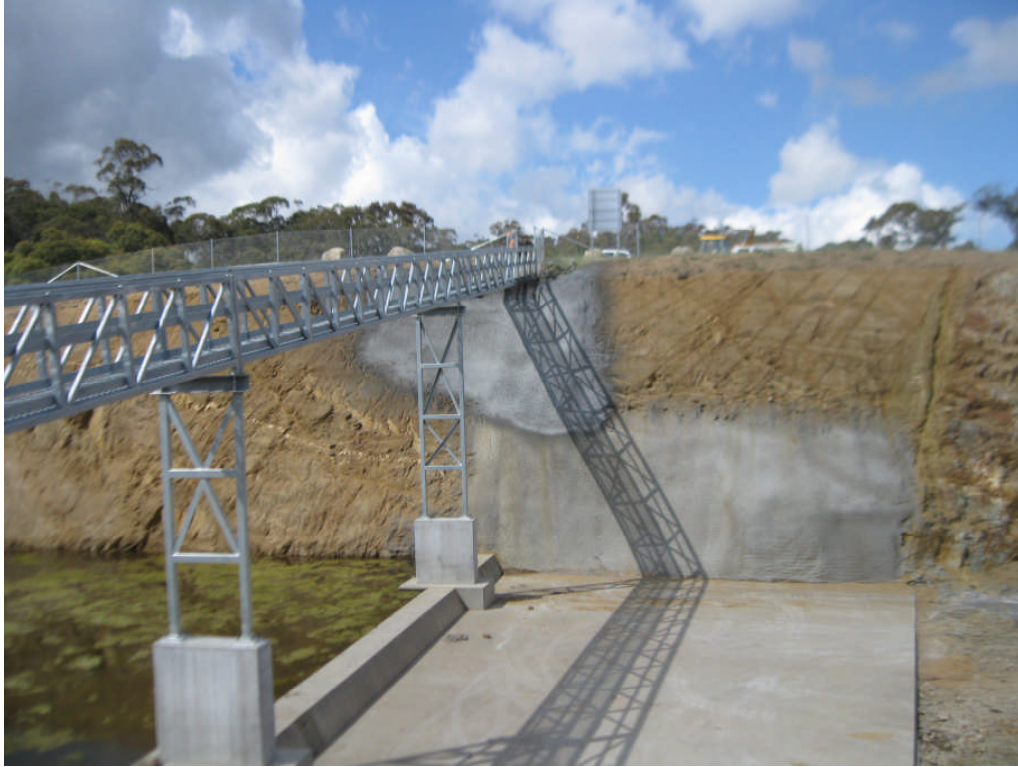
Lake Wallace Dam: Shotcrete anchoring of spillway wall under footbridge
