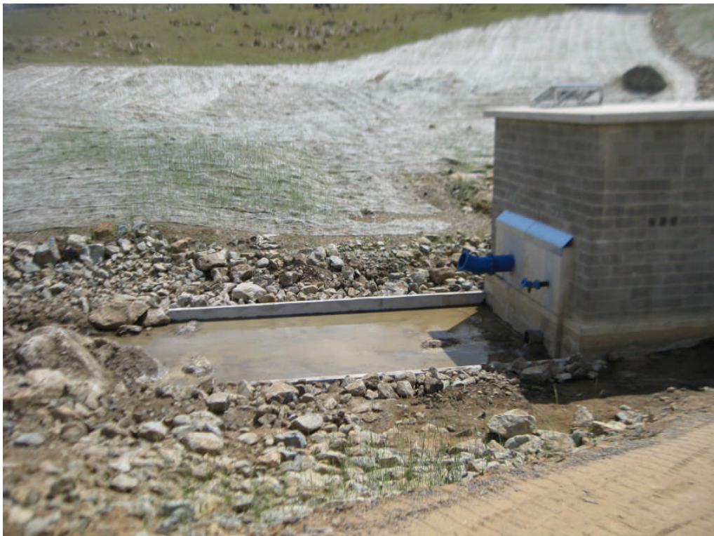
Lake Wallace Dam: Bunded dissipation pad downstream of discharge point
