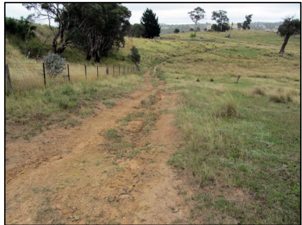
Figure 6-9 Eroded track surface on slope in Lake Wallace block requiring resurfacing and drainage
